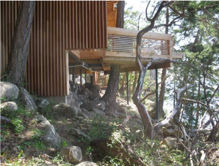
Photo 3. View southeast along DPA showing privacy wall and deck.
