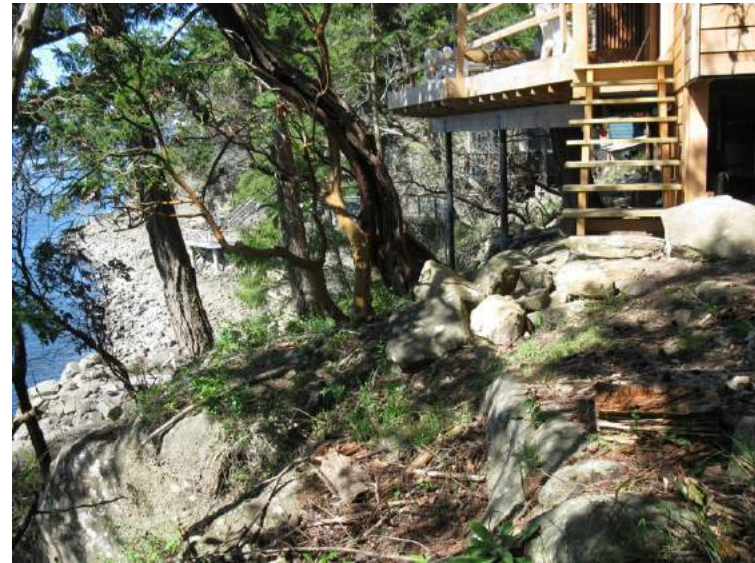
Photo 4. View northwest along DPA showing stairs and steep slope.
