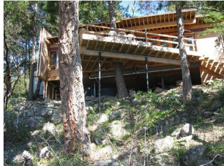
Photo 5. Support posts and Douglas-fir through decking in DPA.
