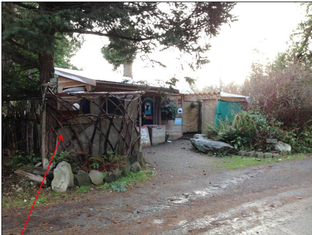
Pergola – Structure 'G'
