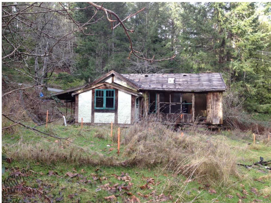
Picture 1: Existing Road House Dwelling Unit (Looking north towards Porlier Pass Rd – Putter Creek runs between road and house)
