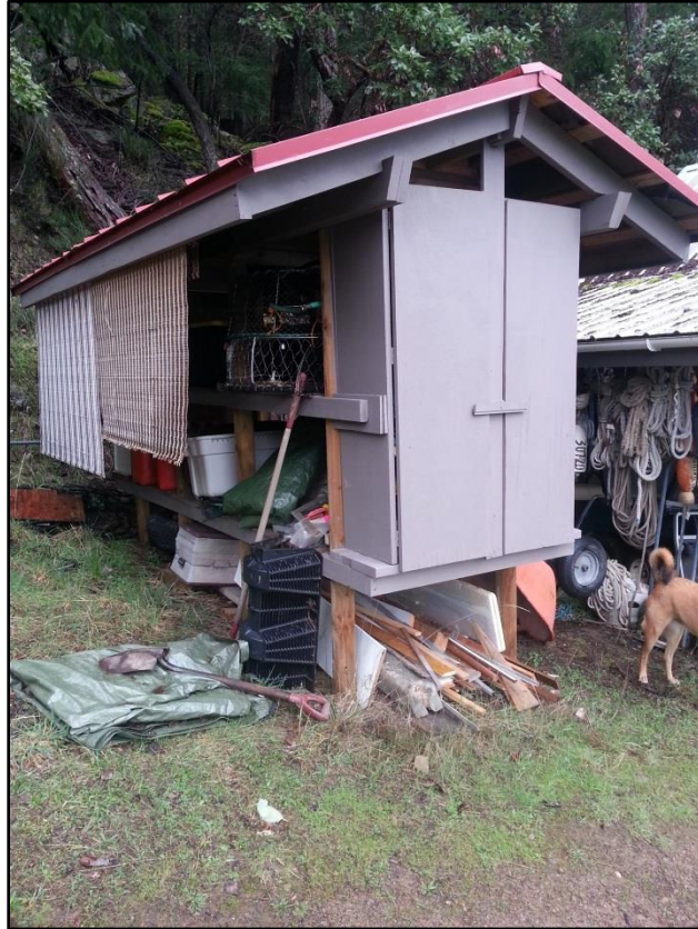
Picture 2: Existing shed – siting variance required (provided by property owner)
