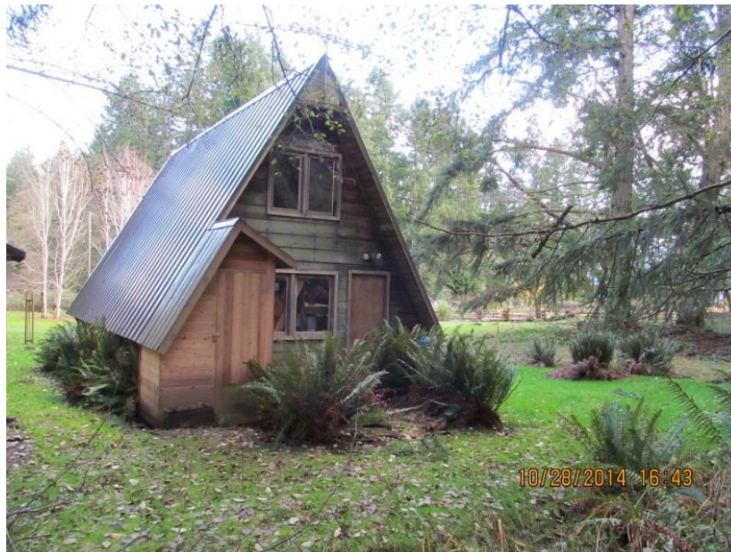
Photo Three: Existing Cottage (Rear and West/Area of Proposed Addition)
