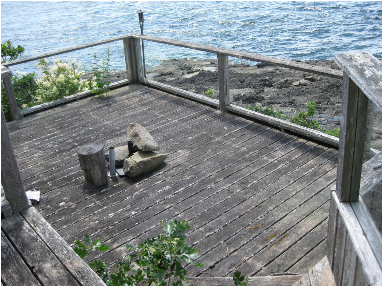
Photo 3 Existing deck in setback area
