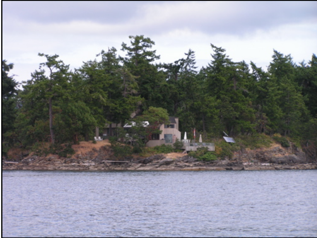
Picture 1 – Existing Single Family Residence
