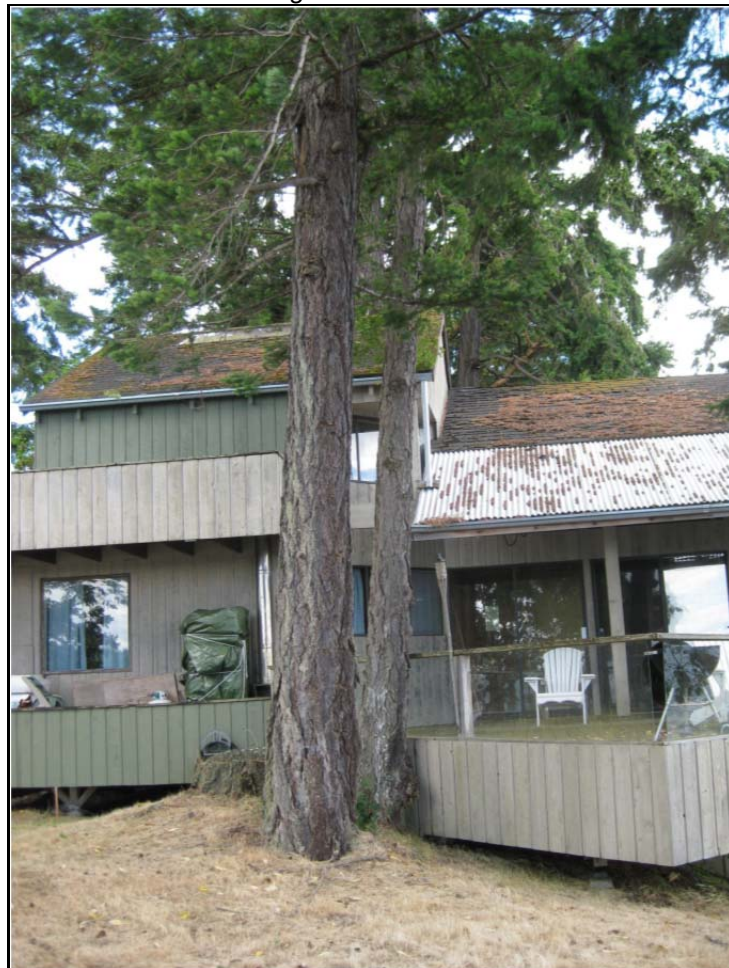
Picture 4 – Douglas-Fir trees to be removed with new construction.
