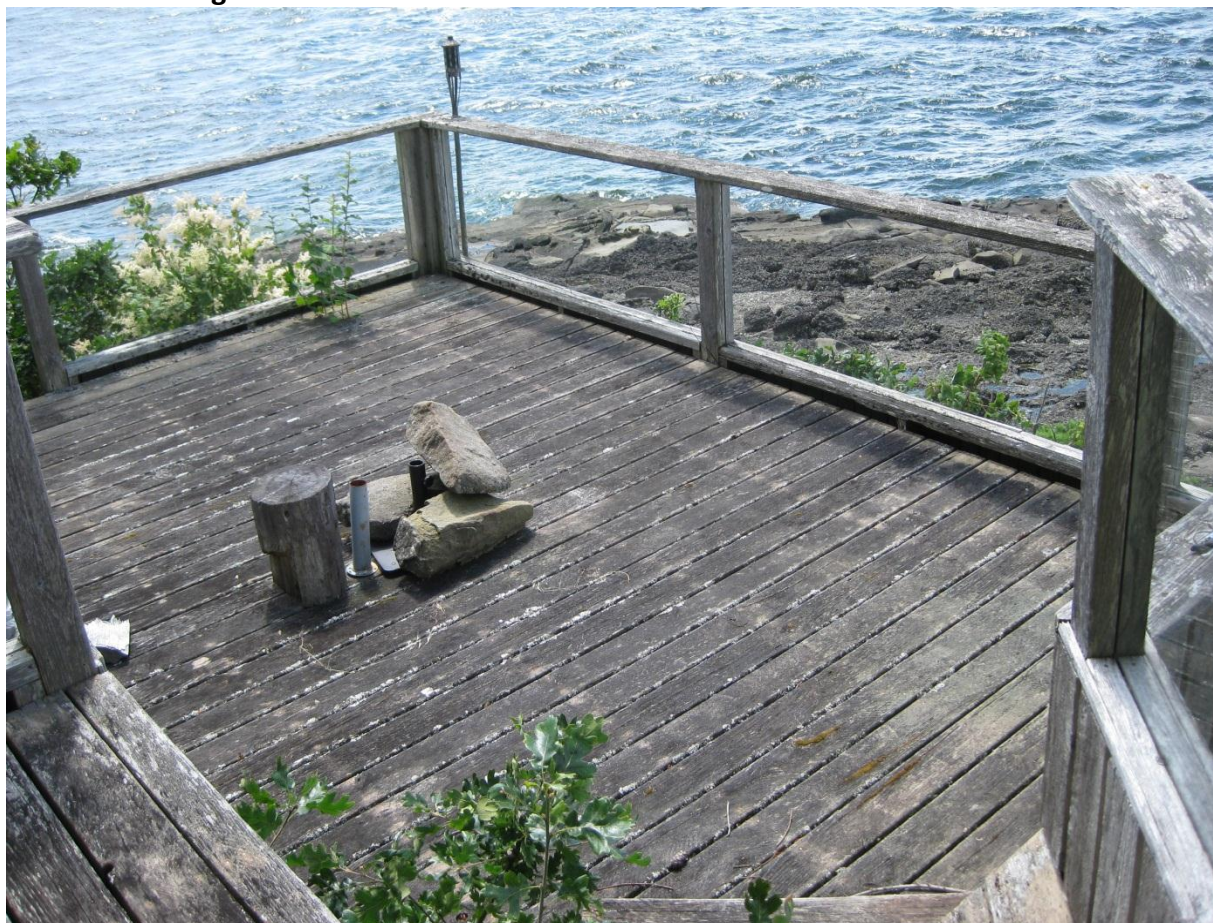
Photo 3 Existing deck in setback area
