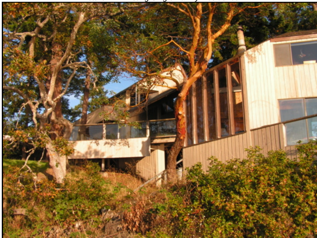
Picture 2 – Existing Single Family Dwelling
