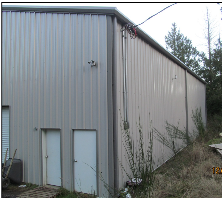
Picture 3 – South Side of Barn
