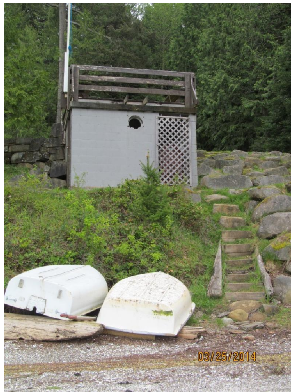
Picture 2: Non-compliant shed and second stairway to beach
