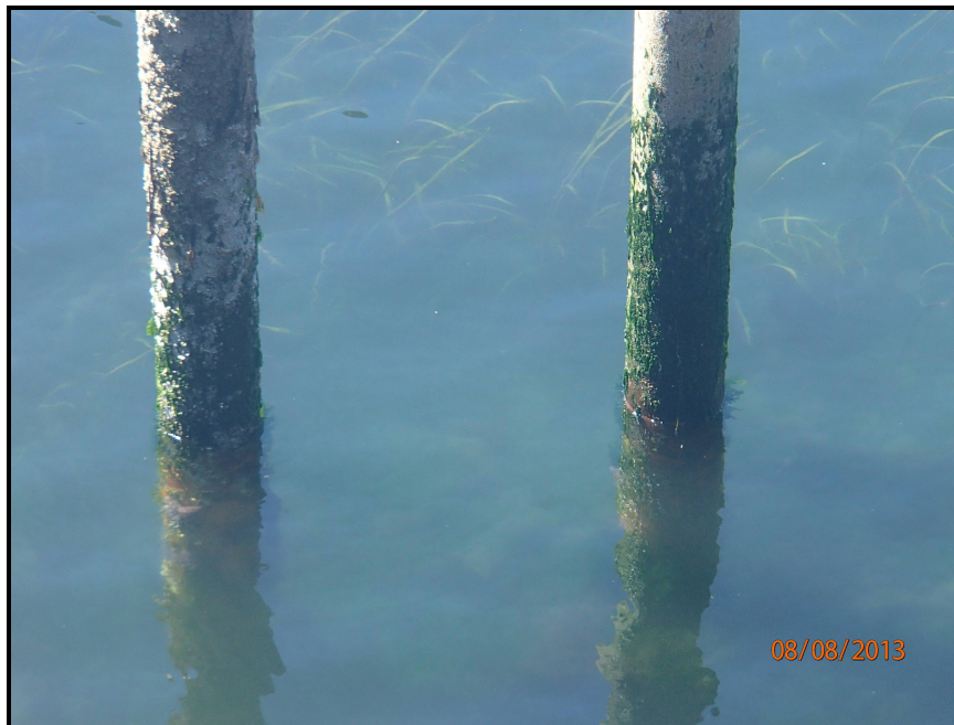
Photograph 2. Close-up of eelgrass between the pilings closest to shore.
