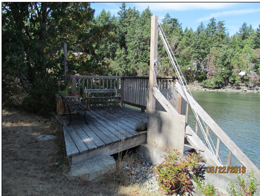
Picture 3: Deck and stairs on retaining wall
