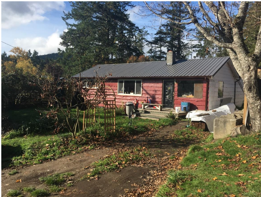
PHOTO 1. EXISTING DWELLING AT 60 MADRONA ROAD
