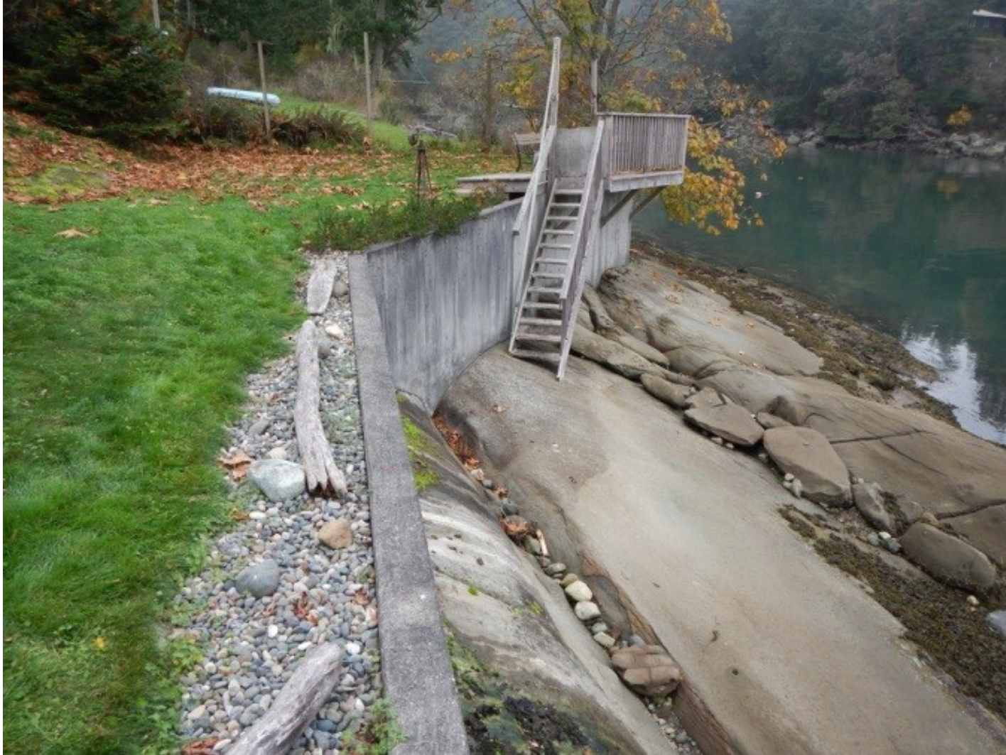
Figure 3. Photo along the top of the seawall. Note the absence of riparian vegetation.
