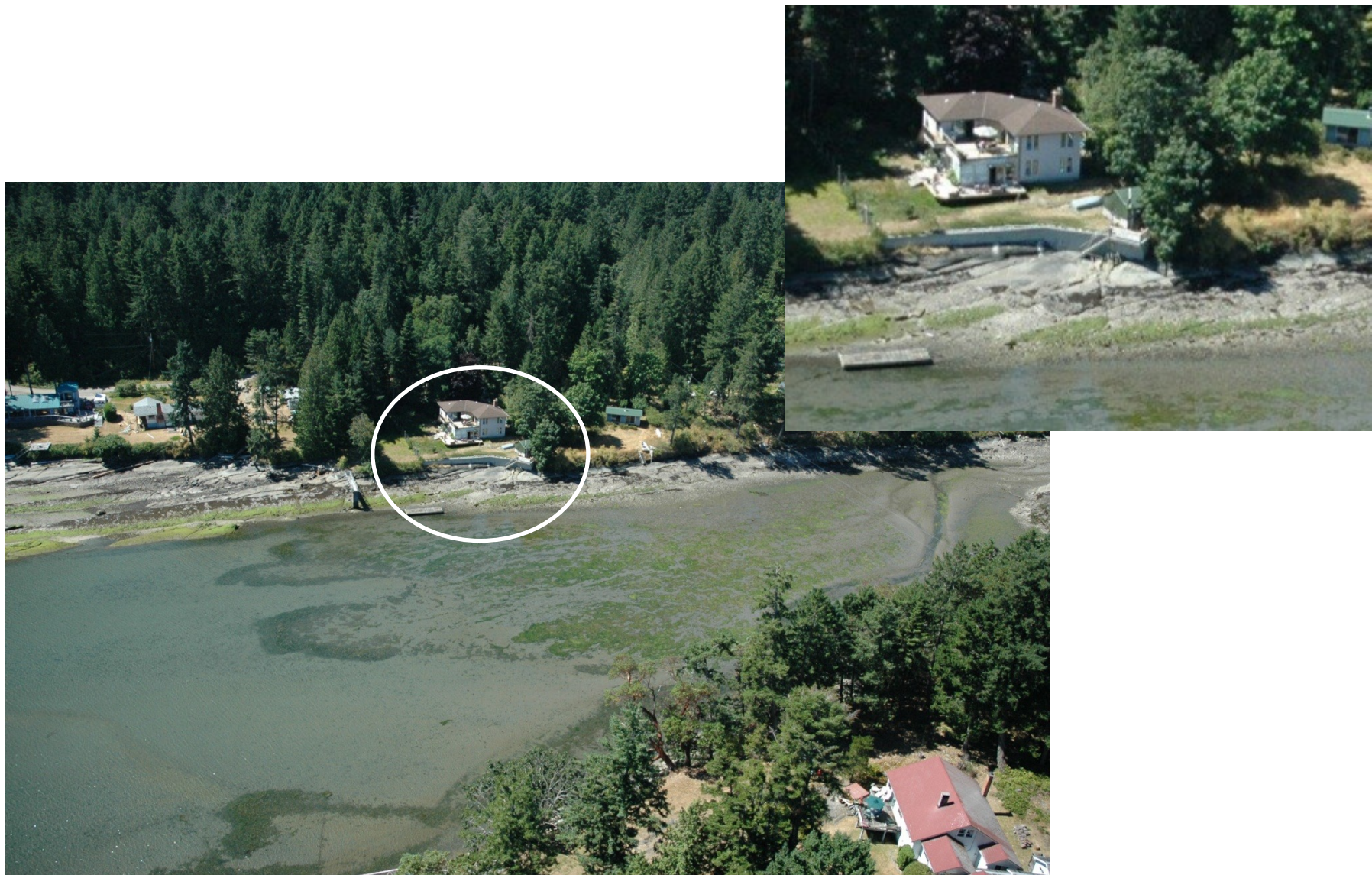
Figure 2. Aerial photo from the July 2005 ShoreZone survey showing 260 Cayzer Road property and the associated seawall. The photo was shot at a near “zero” tide.
