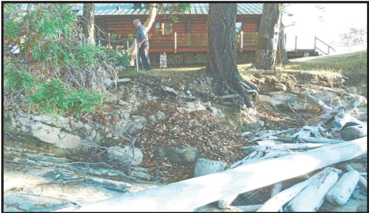
Photograph 2: Approximate north view of western extent of proposed bank stabilization works.
