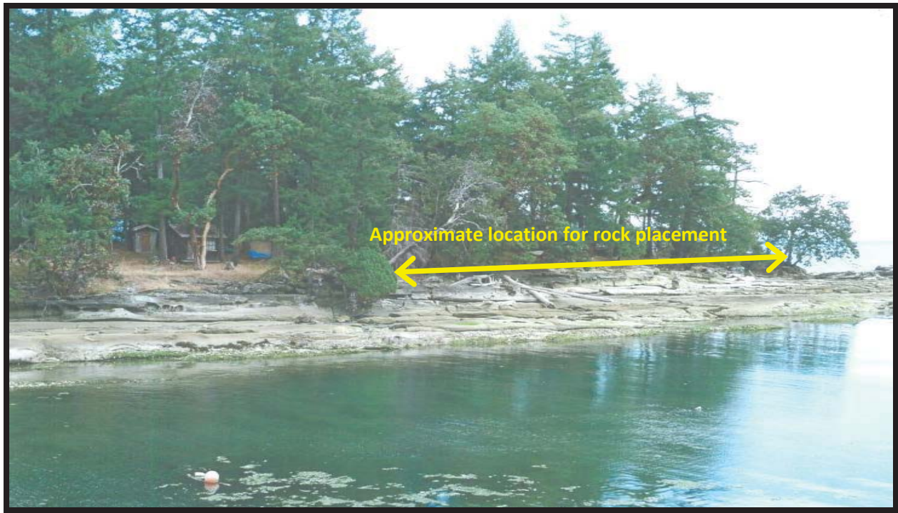
Photograph 1: Approximate northeast view of location of proposed bank stabilization works.
