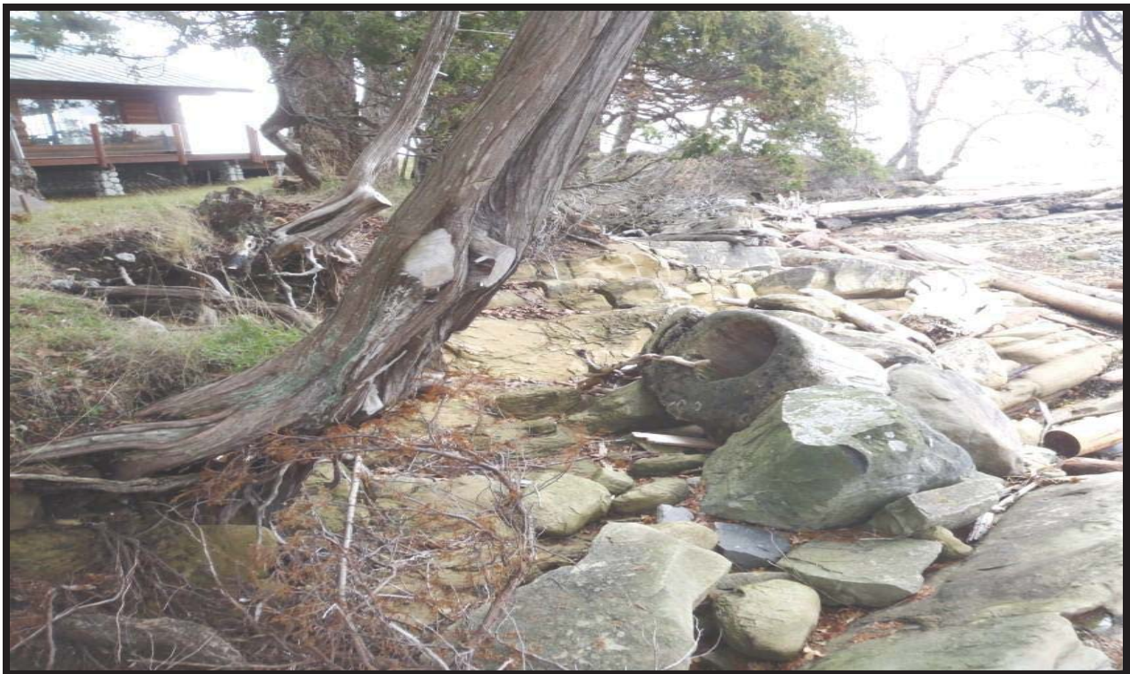
Photograph 6: Approximate east view along the top-of-bank of proposed bank stabilization works.
