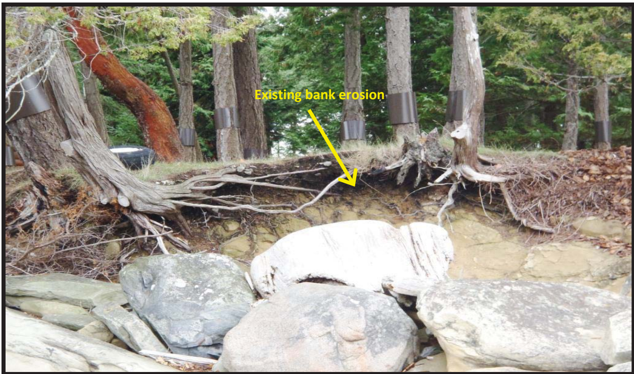
Photograph 4: Approximate northwest view of the central portion of proposed bank stabilization works.
