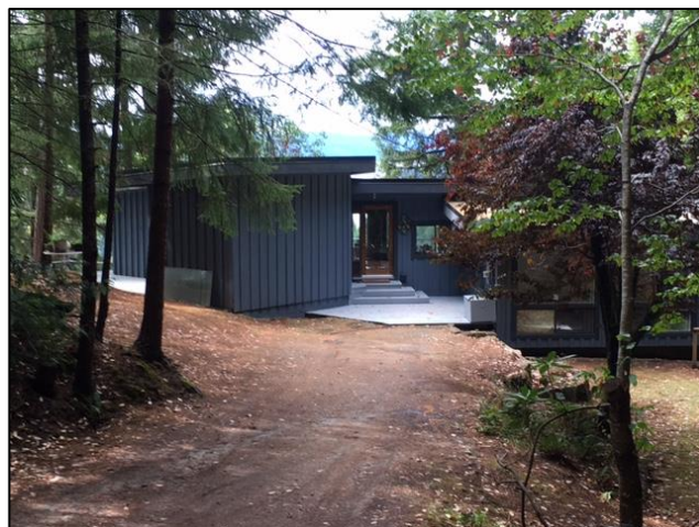
Image 6: View of dwelling unit from driveway
