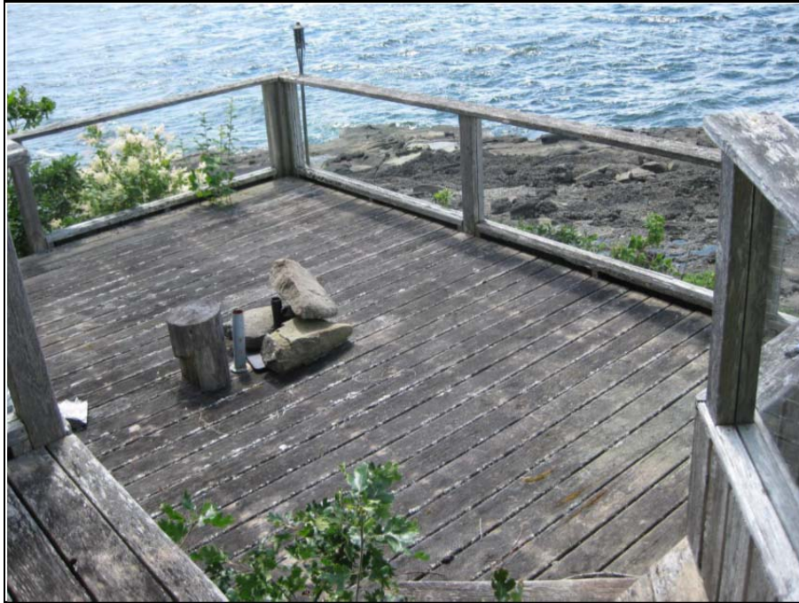
Picture 3 – Existing deck within setback to the sea
