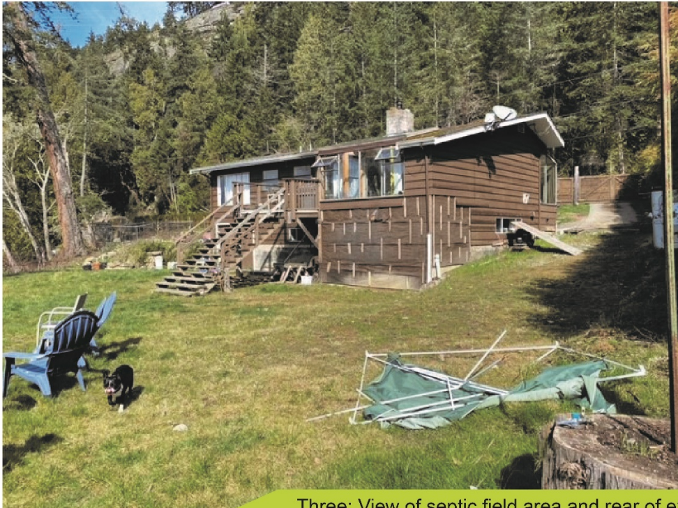
Three: View of septic field area and rear of existing dwelling
