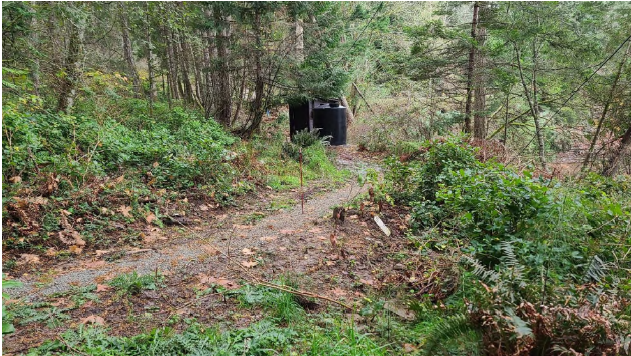
Photo 1: Shows the water tank and pumphouse along with the access path from driveway.
