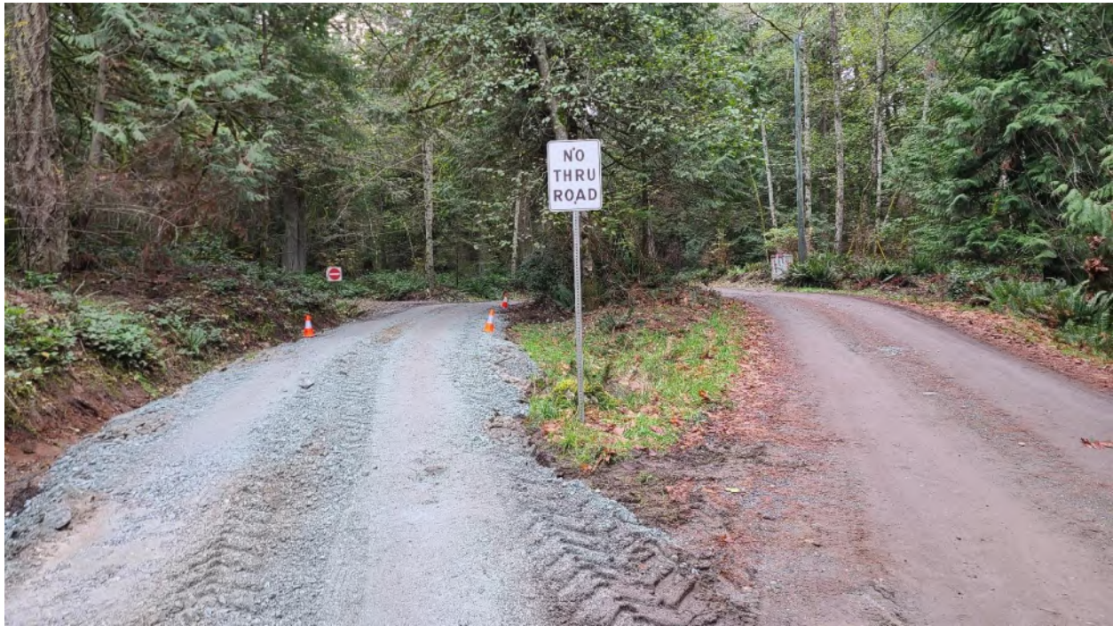
Photo 5: Looking up Gardner Road from Sturdies Bay Road. The pipe/cable is buried under the fork on the left and then crosses over to the well head just beyond the mailboxes in the background.
