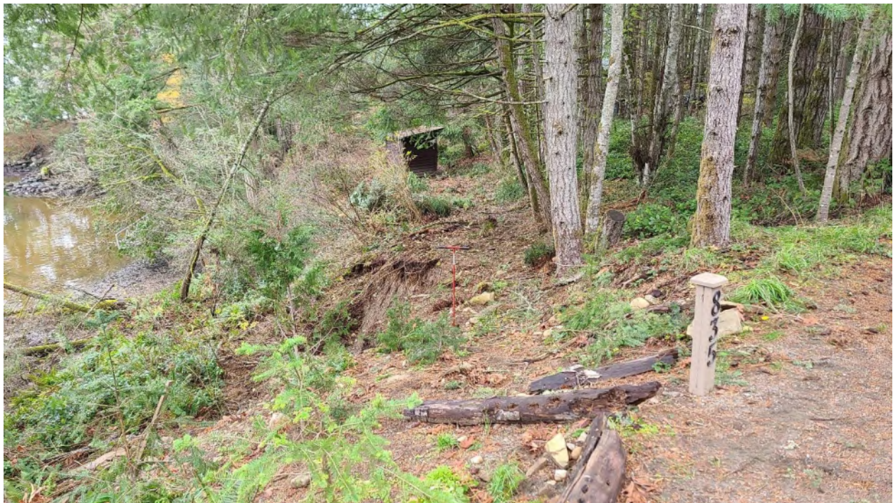
Photo 2: Shows the pumphouse and pipe/cable route from the edge of Sturdies Bay Road.
