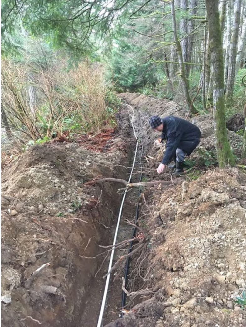
Photo 1 – Water line and power line construction trench.
