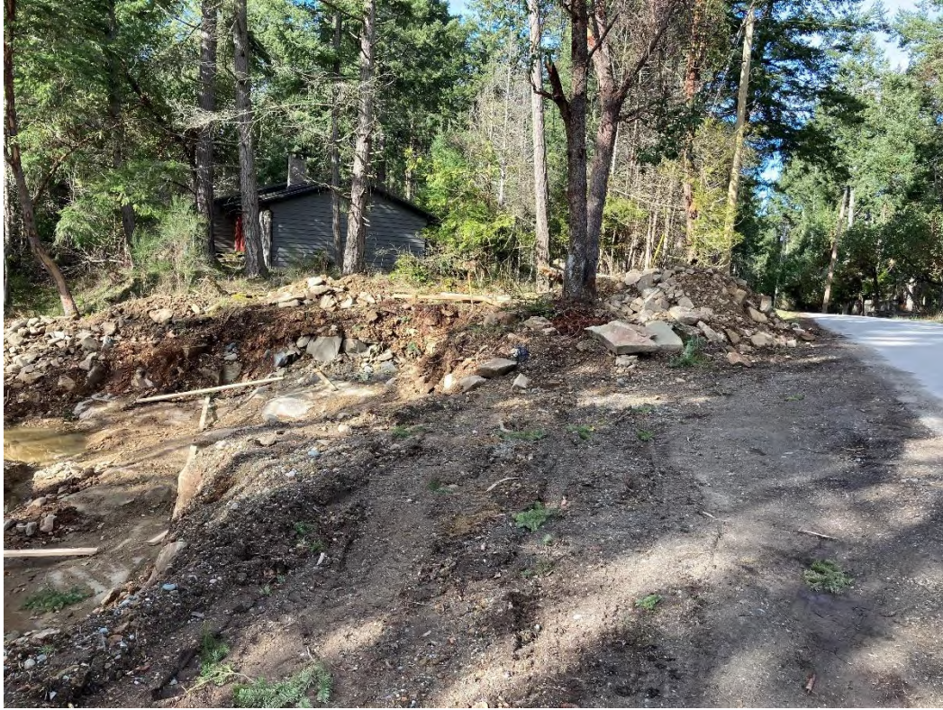
LOOKING WEST TOWARDS NEIGHBOURING HOUSE AND CORNER OF WORKSHOP/MAEKERY LOCATION (AREA FOR POTENTIAL FENCE)
