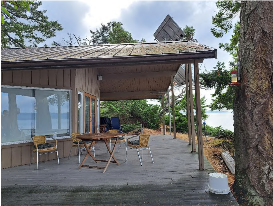
LOOKING SOUTHEAST (DWELLING, DECK, SOLAR PANEL)
