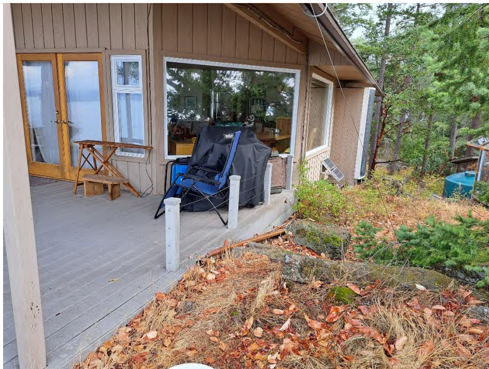
LOOKING NORTHEAST (DWELLING, DECK, AND INTERIOR LOT LINE)
