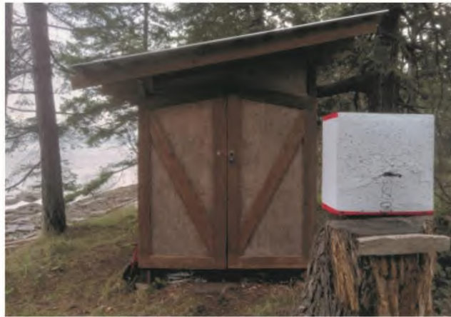
Accessory shed (looking east)
