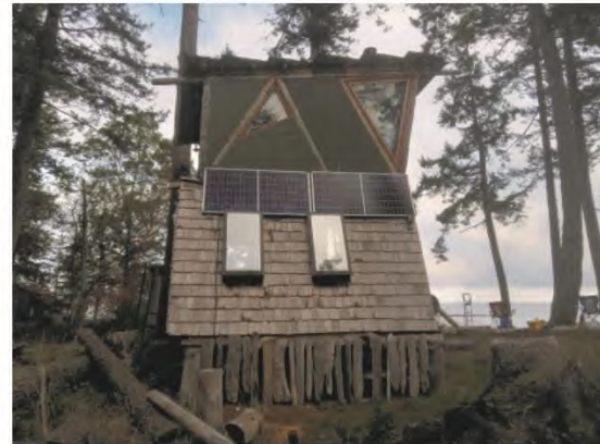
Accessory building (looking northwest)
