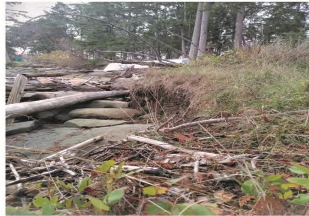
View east along foreshore
