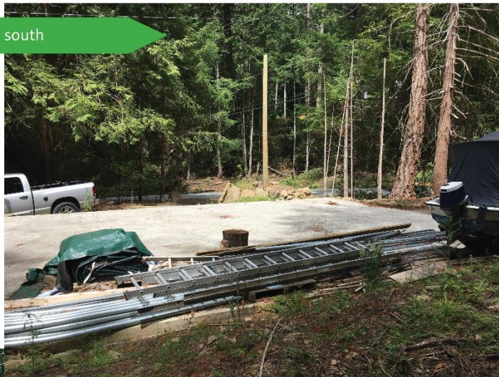
North access on Porlier Pass Rd.
