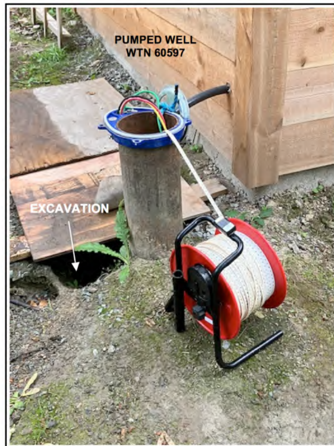
Figure 4. Photo of wellhead of pumped well taken June 11, 2024 showing excavated area to be filled around the well casing.
