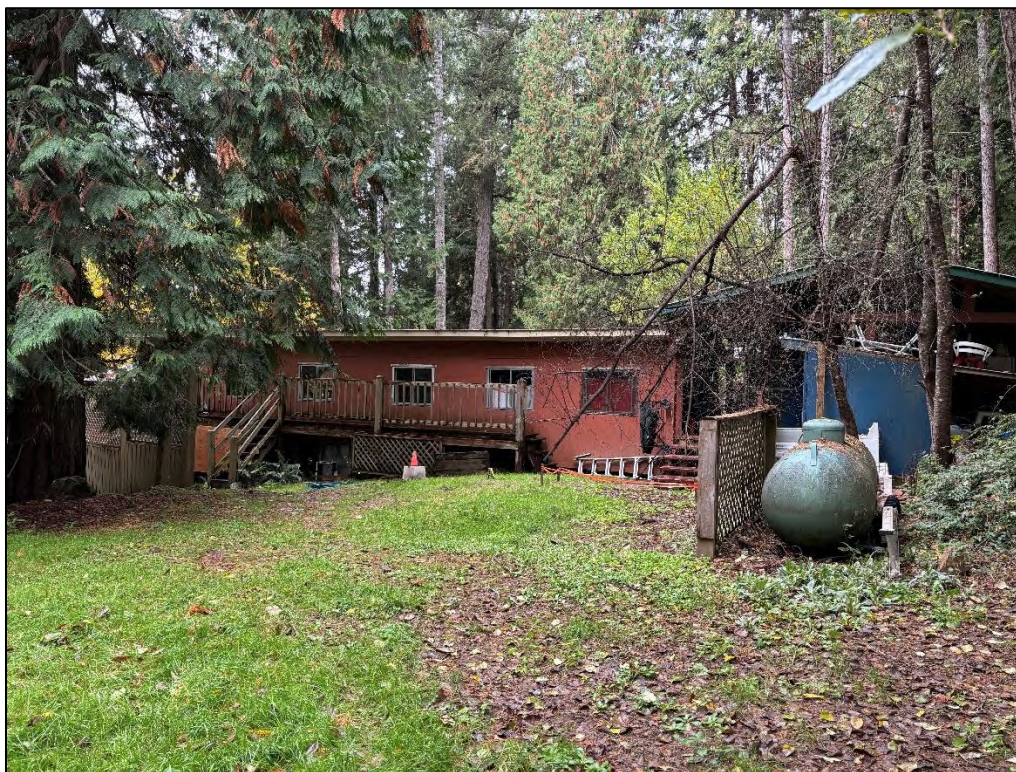
LOOKING WEST TOWARDS EXISTING BUILDING
