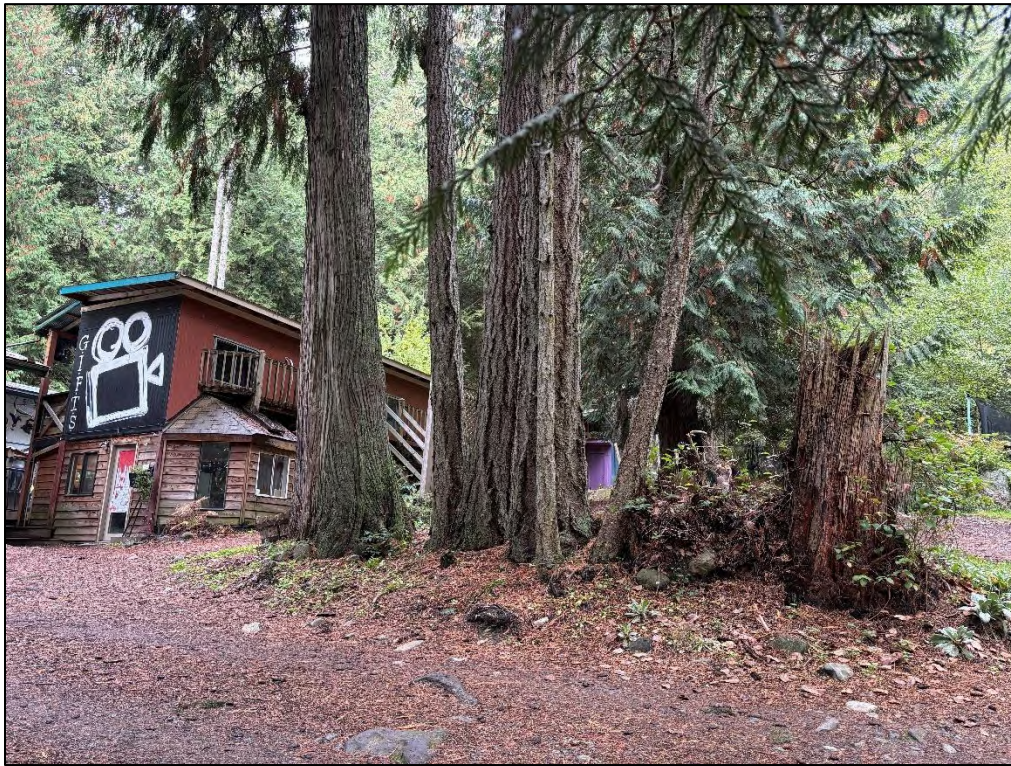
LOOKING NORTH TOWARDS EXISTING BUILDING CURRENTLY USED FOR COMMUNITY HOUSING
