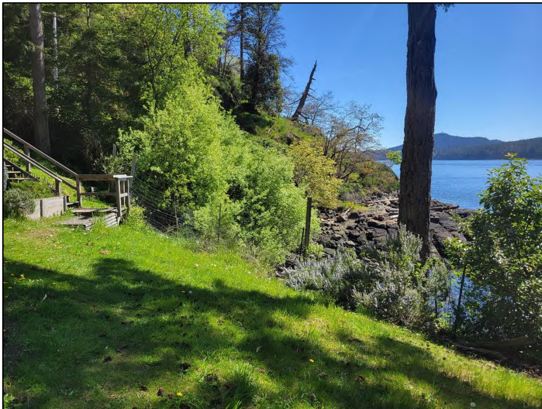
EXISTING STAIRS AND LANDING, AND APPROXIMATE LOCATION OF NEW ABSORPTION FIELD, LOOKING EAST
