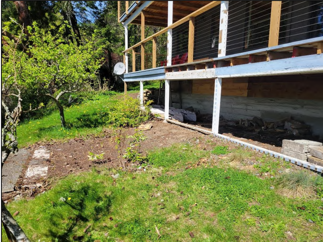
DECK AND APPROXIMATE LOCATION OF NEW ABSORPTION FIELD, LOOKING WEST
