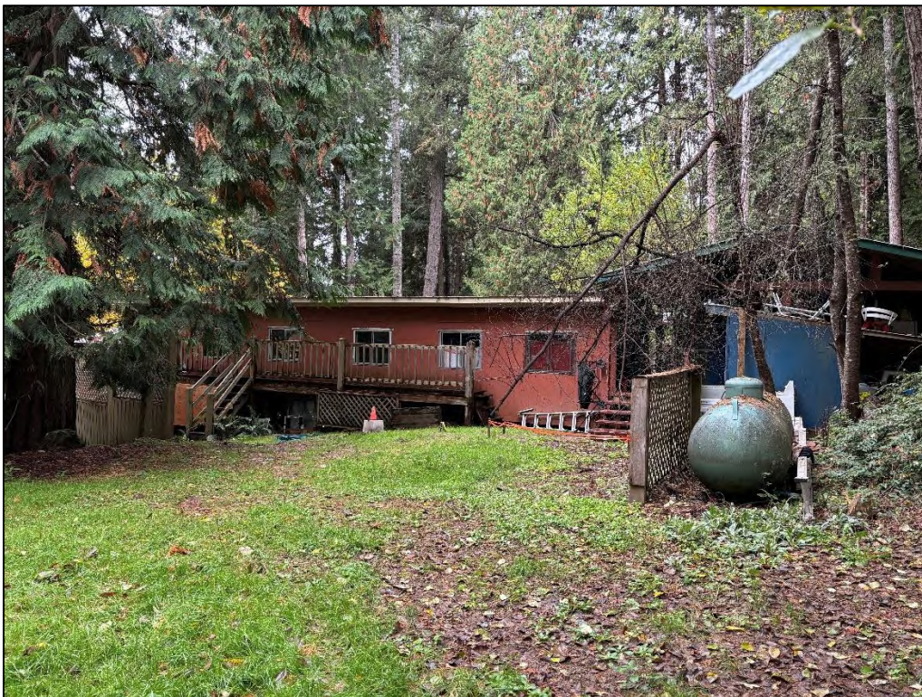
LOOKING WEST TOWARDS EXISTING BUILDING
