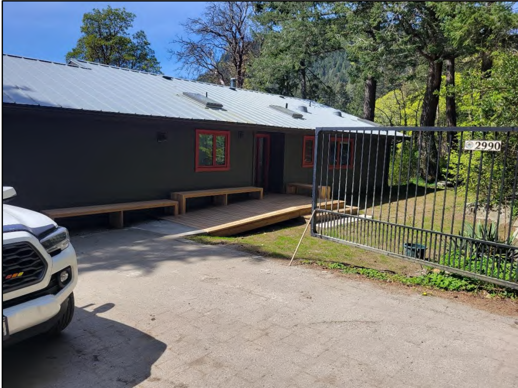
PARKING AREA, LOOKING SOUTH-WEST
