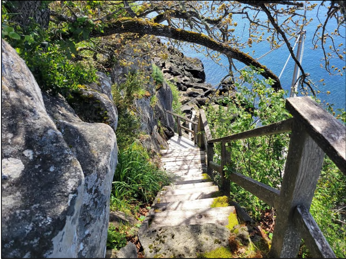
EXISTING STAIRS AND LOWER LANDING, LOOKING SOUTH
