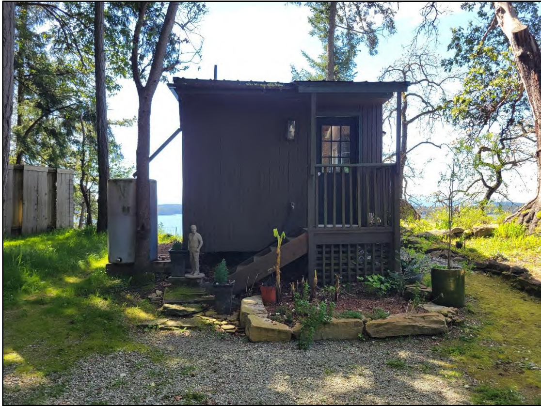
ACCESSORY CABIN, LOOKING WEST
