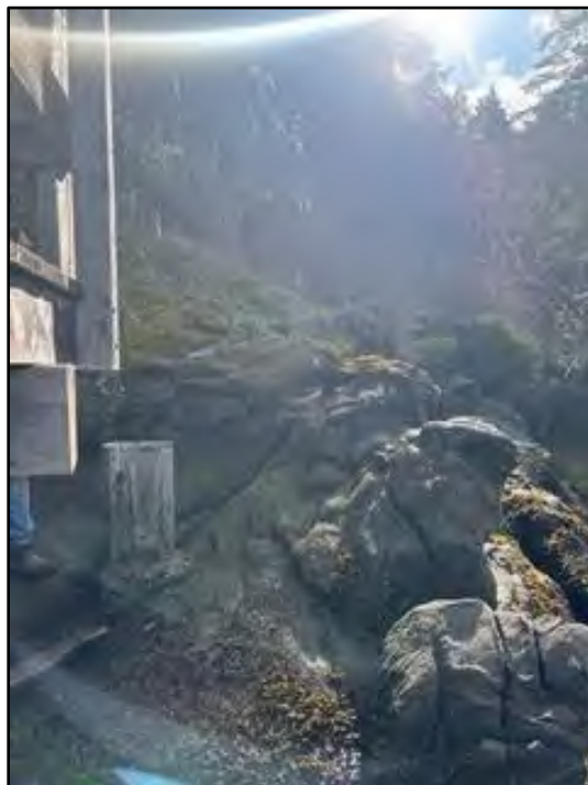
EXISTING CONCRETE PILING
