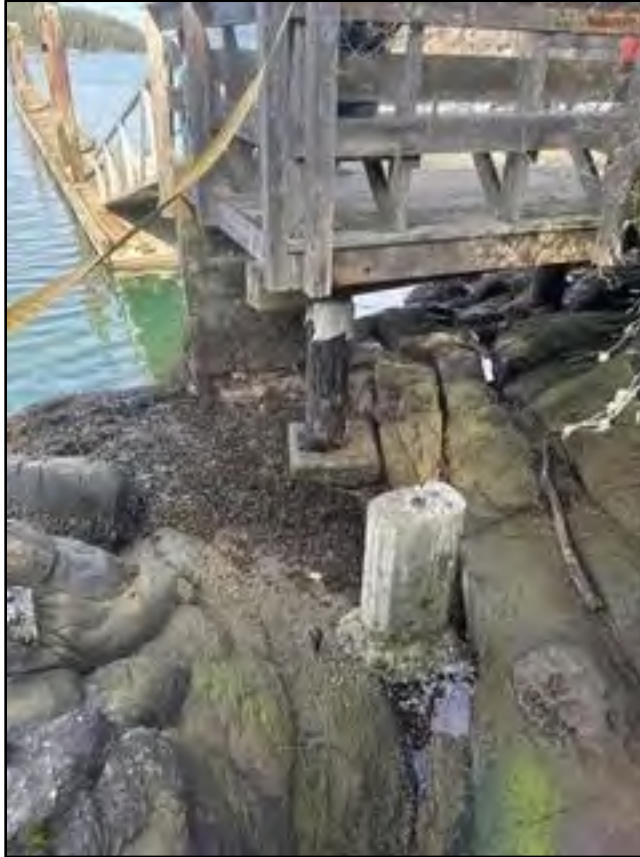
EXISTING CONCRETE PILING AND DOCK
