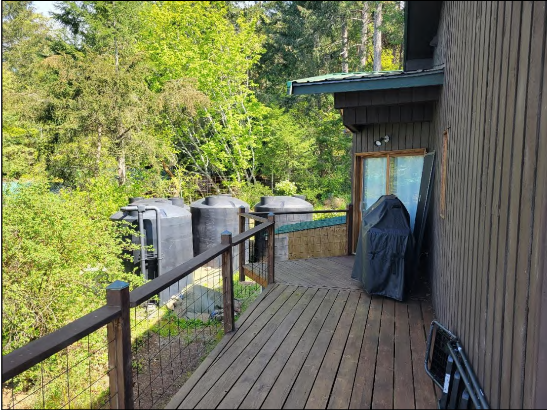
NORTH SIDE OF DWELLING AND DECK LOOKING EAST
