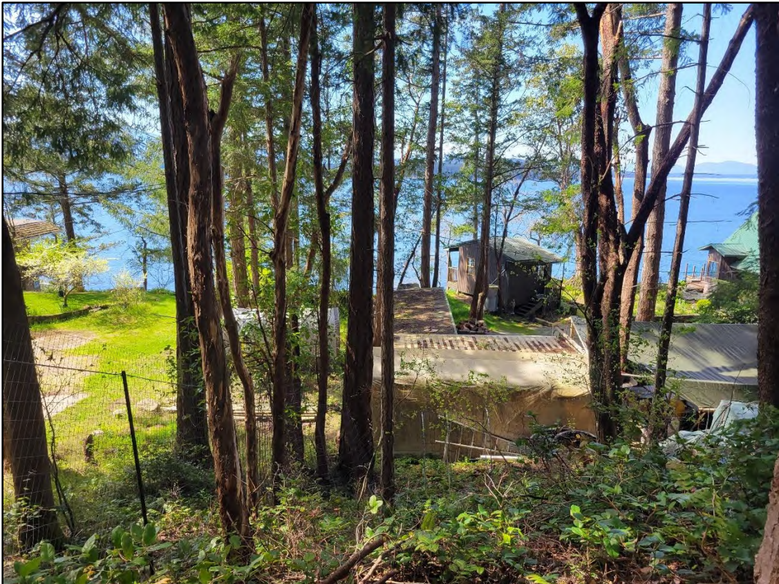
WOOD STORAGE SHED AND CONTAINER, LOOKING WEST
