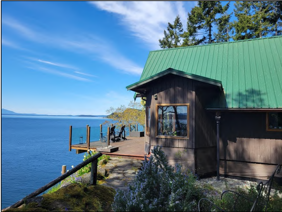
EXISTING DECK AND DWELLING, LOOKING NORTH
