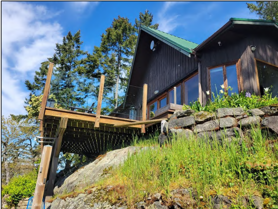
EXISTING DECK AND DWELLING, LOOKING NORTH
