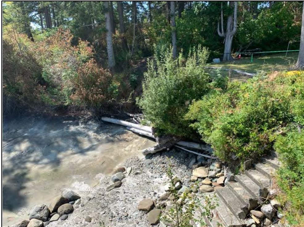
PROPOSED SEAWALL LOCATION AND EXISTING STAIRS, LOOKING SOUTH ACROSS INLET
