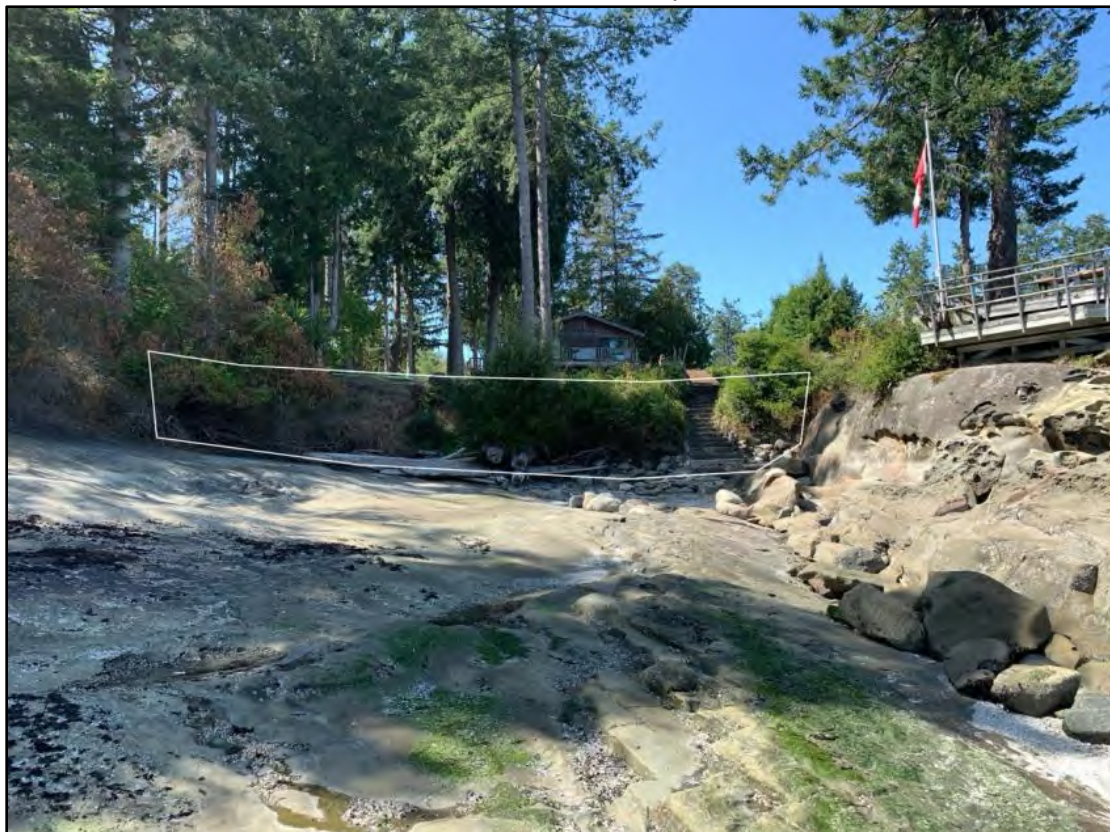
APPROXIMATE SEAWALL FOOTPRINT, LOOKING WEST
