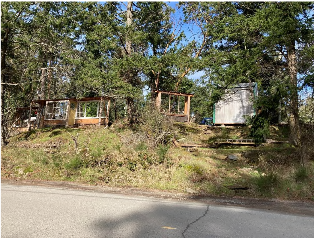
STRUCTURES LOCATED WITHIN FRONT LOT LINE SETBACK (LOOKING NORTH FROM STURDIES BAY ROAD)
