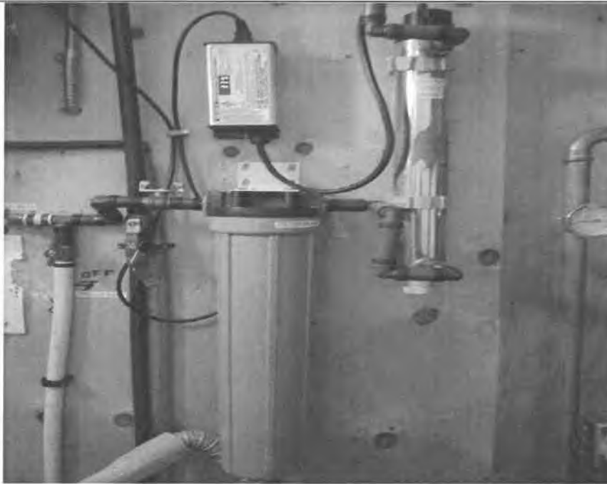
Photo 1. System includes a Controller, a large Filter (Blue Container) and UV Light (Stainless Steel tube) to treat and filter the well water.
