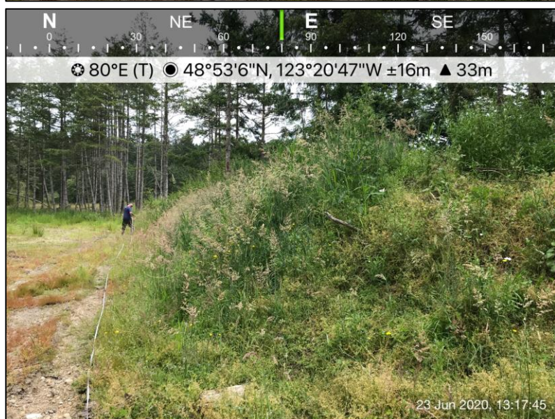
Photo 3: Large berm at the south boundary of landing area. Fully overgrown with weeds and other vegetation
