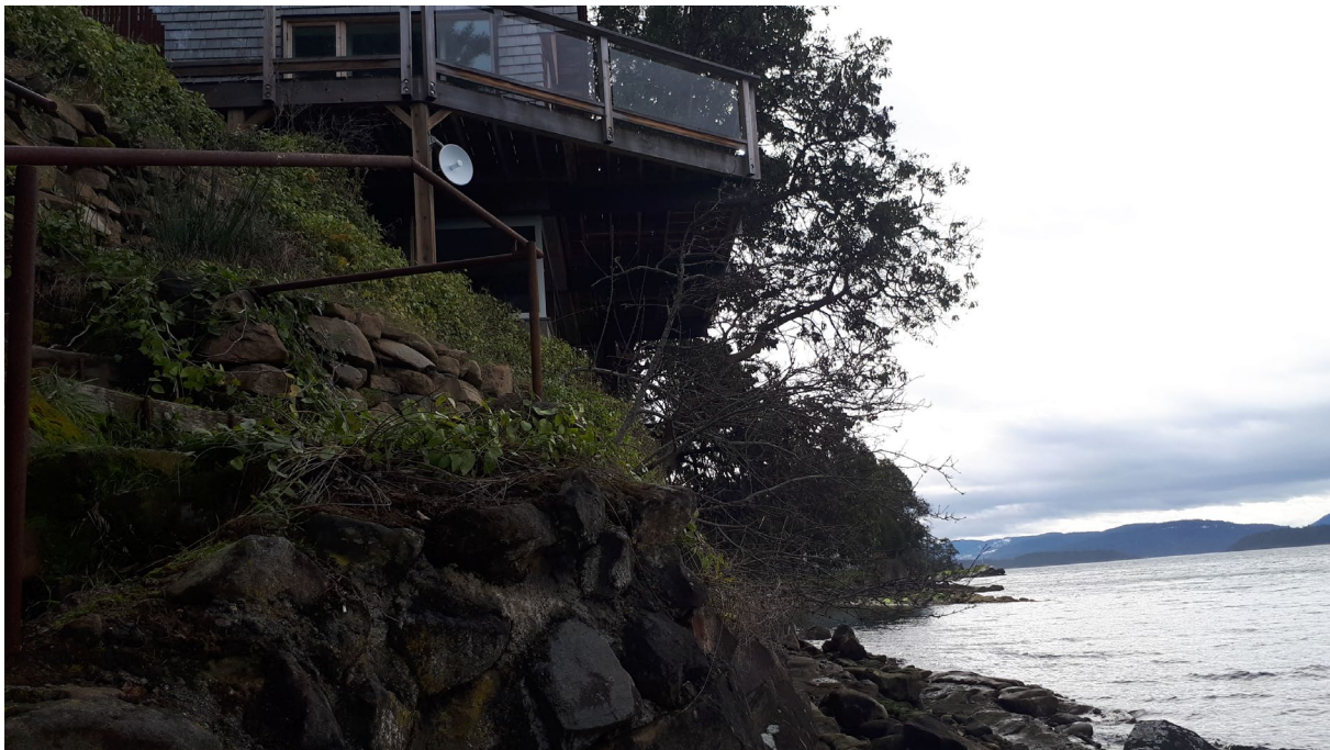
Plate 4. Natural boundary of the sea at base of current dwelling at 21455 Porlier Pass Rd., Galiano Island, BC.
