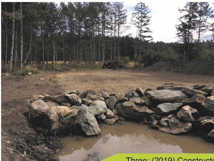
Three: (2019) Constructed pond with landing and berm beyond
