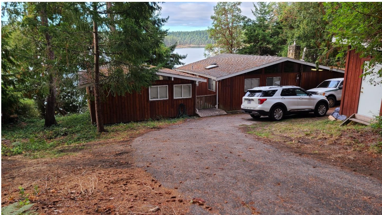
Photo 6: Shows the existing main dwelling, breezeway, annex, driveway and shed. The 15m DPA2 setback roughly parallels the back of the structures (edge closest to driveway). The small diameter Douglas-fir in line with the left (east) side of the annex will be removed but is outside of the DPA2 setback. The arbutus tree on the far left of the photo will not need to be removed.
