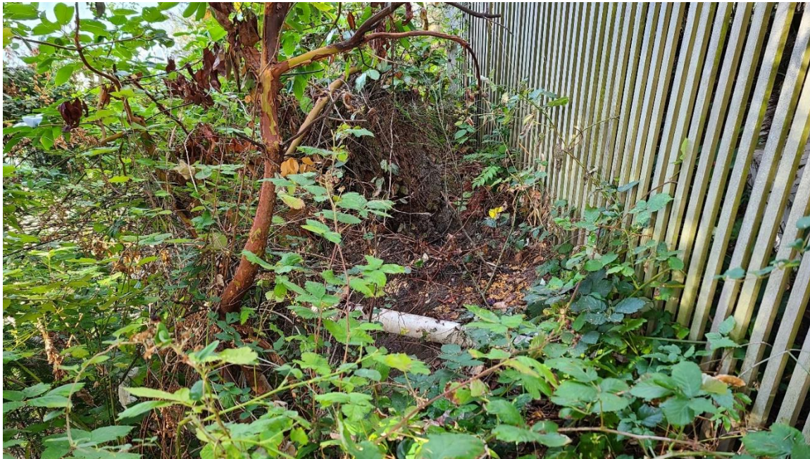
Photo 8: The white pipe under the vegetation in the foreground is the perimeter drainage.
