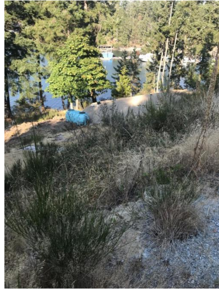
Septic installation immediately northwest of subject property
