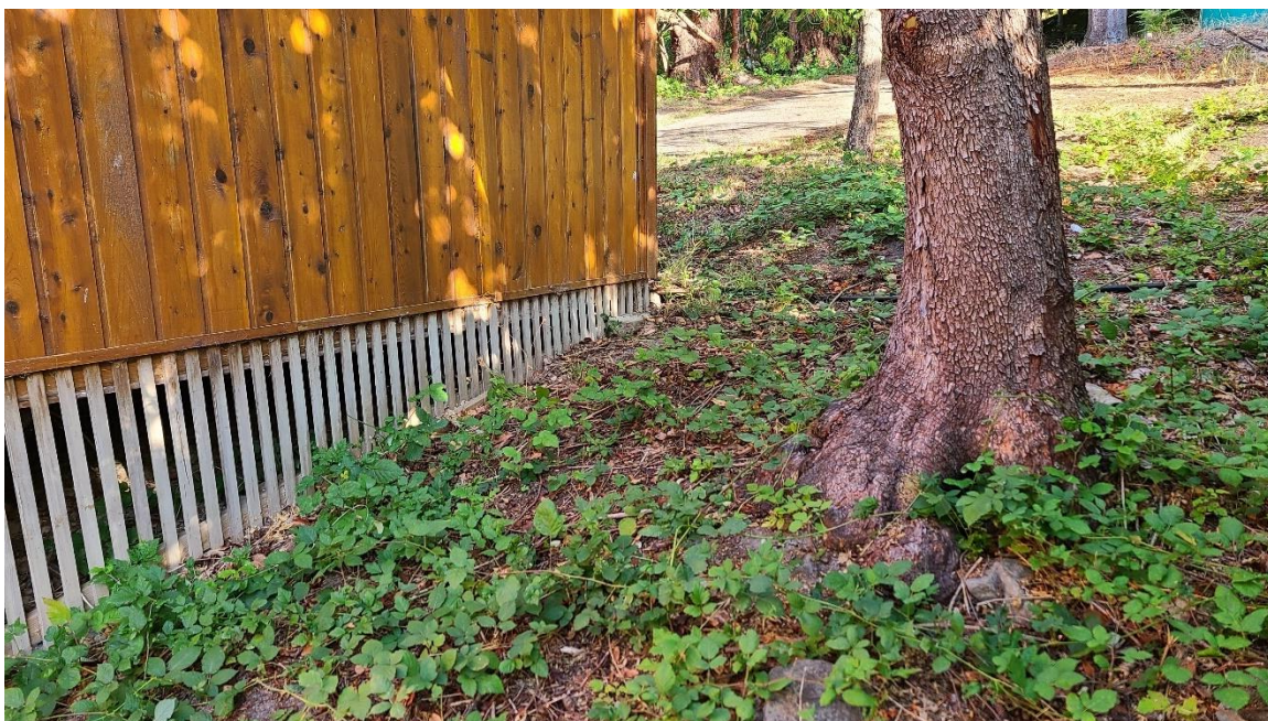
Photo 9: Shows the proximity of the arbutus tree to the existing building.
