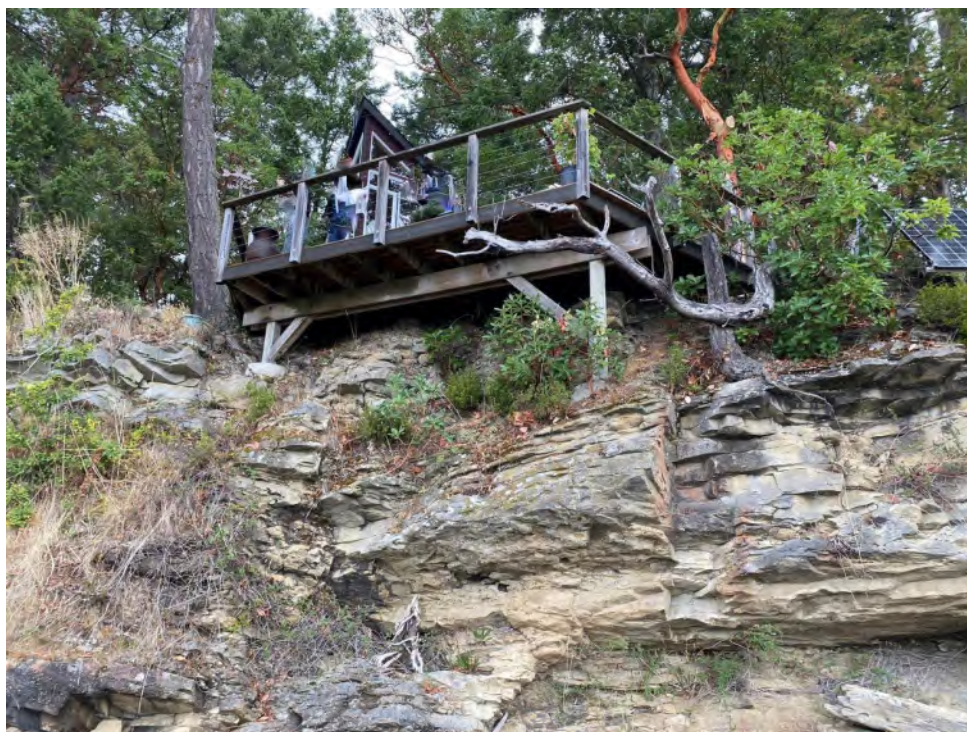
Cantilevered Lower Deck
