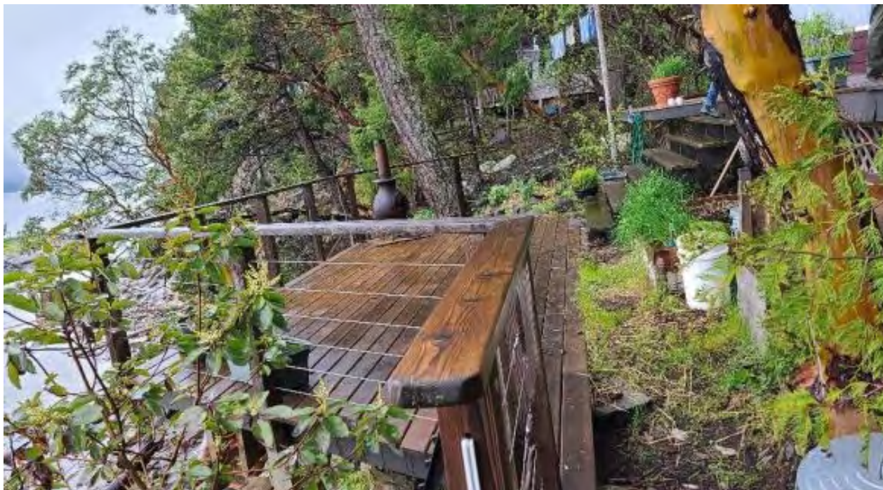
Picture of Existing Lower Deck (Photo from Environmental Assessment prepared Keith Erickson)
