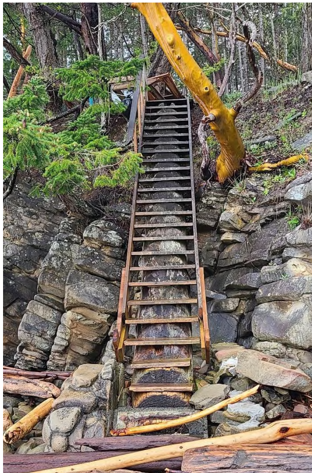
Photo 6: Shows the cedar log beam along with the constructed treads, stringers and railing (left). The upper landing (top right) and the portion of the steps that have been removed by the owner in 2022 (right).
