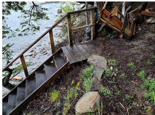
Photo 6: Shows the cedar log beam along with the constructed treads, stringers and railing (left). The upper landing (top right) and the portion of the steps that have been removed by the owner in 2022 (right).
