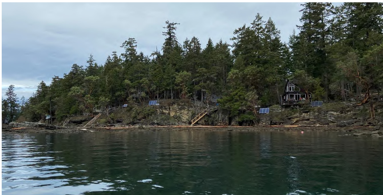
LOOKING NORTHEAST (MULTIPLE WISE ISLAND PROPERTIES WITH STAIRS AND SOLAR PANELS)
