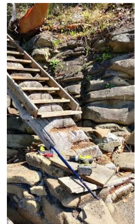
Photo 6: Shows the cedar log beam along with the constructed treads, stringers and railing (left). The upper landing (top right) and the portion of the steps that have been removed by the owner in 2022 (right).
