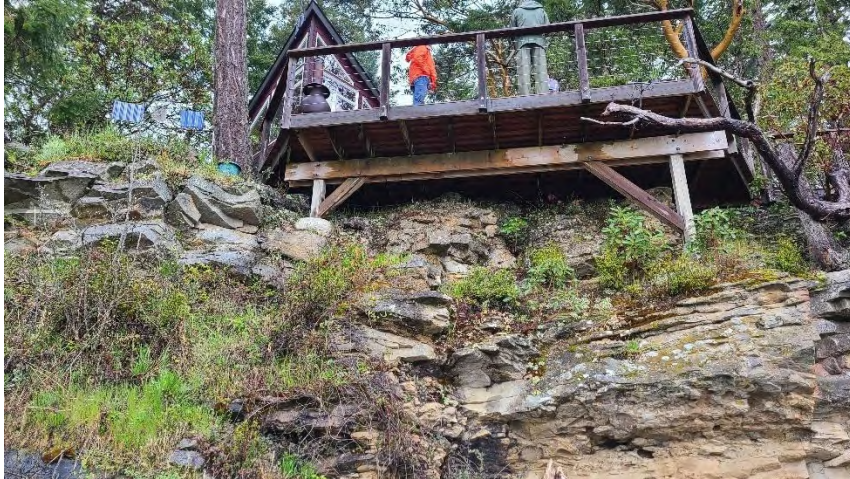
Photo 7: Shows the lower deck from below, cantilevered out over the shoreline cliff.
