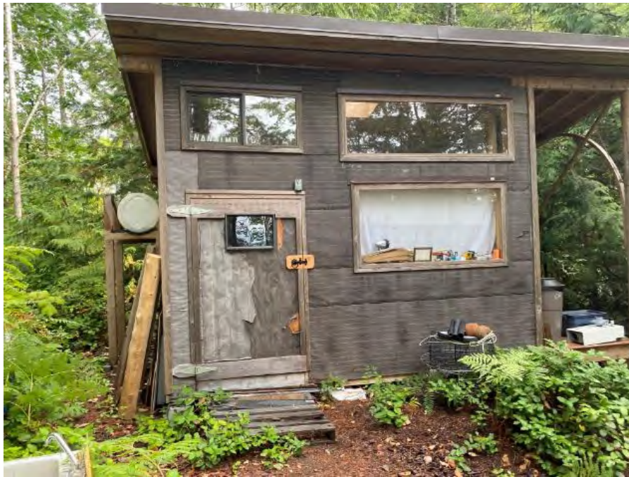
Work shed (taken Aug 31, 2023)
