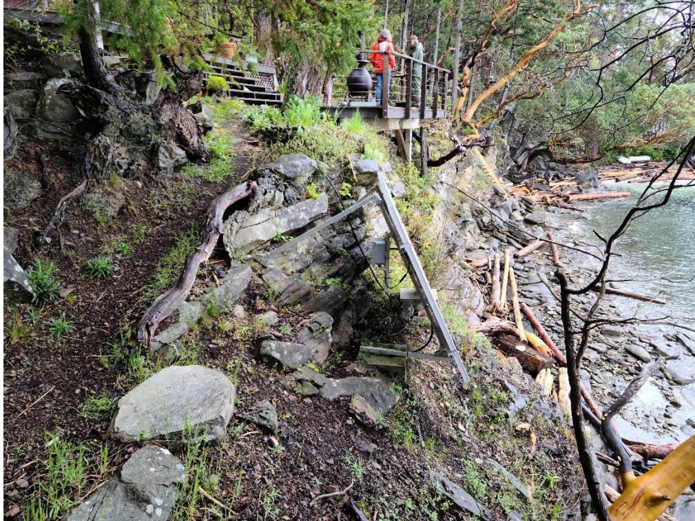
Photo 2: Looking from west to east across the crest of the slope. The footpath from the lower deck to the upper landing of the marine access stairs (photo taken from landing) is seen on the left of the photo.
