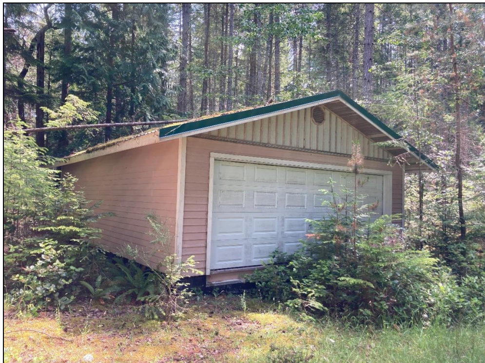
BUILDING (WITH NO POWER OR WATER)
