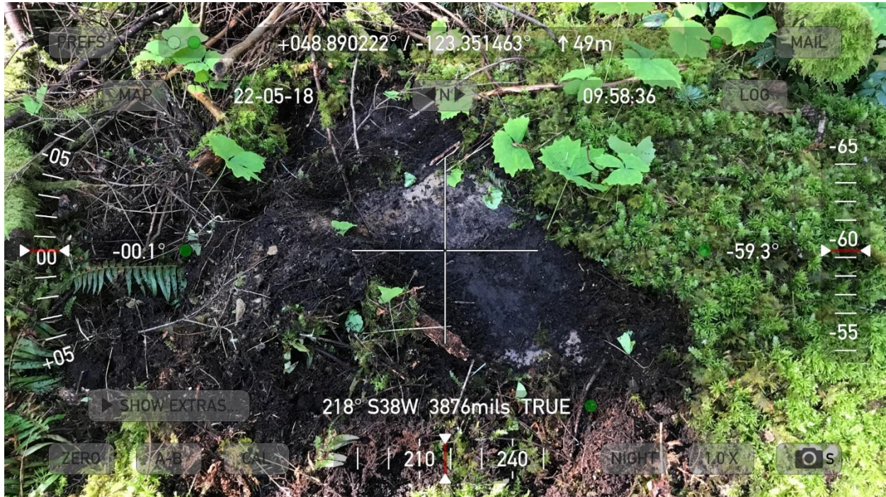
West Mid-Level Bench – Test Pit 5. Example of Bedrock Structure Blocking Ground Water Flow in the SE 26 meters of Inspected Area.
