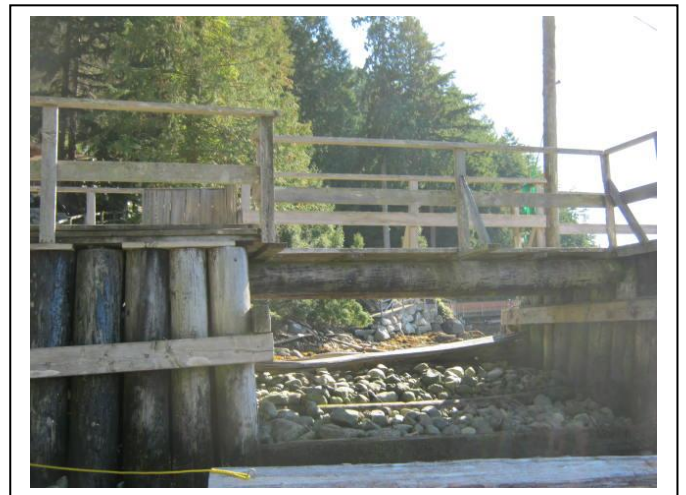
Foreshore structure impeding sediment flow. Photo: RC de Graaf
