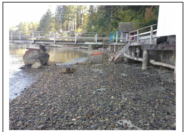
Foreshore structures impeding sediment delivery and flow along beach surface. Photo: RC de Graaf
