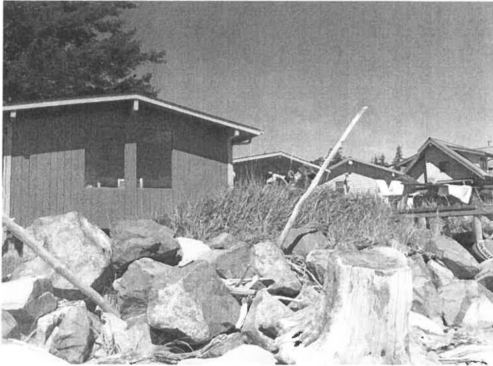
Photograph 3: Breakwater structure found east of the area of proposed development.
