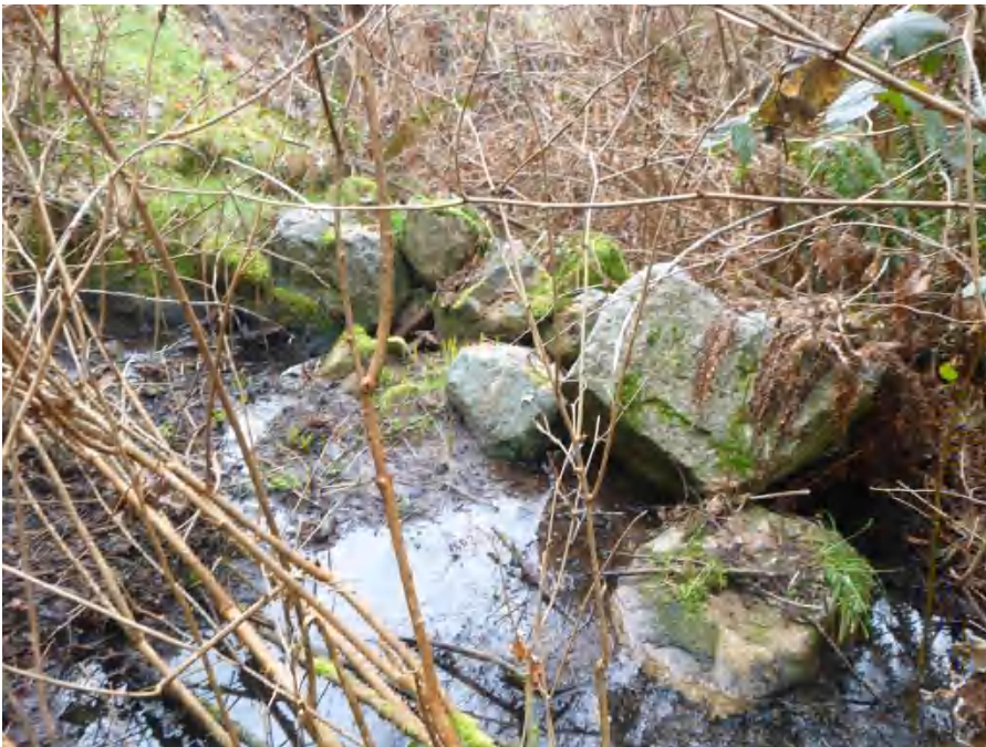
Boulders obscuring the stream channel (potentially from a failed retaining wall) on tributary 1 immediately upstream of the West Bay Road crossing.
