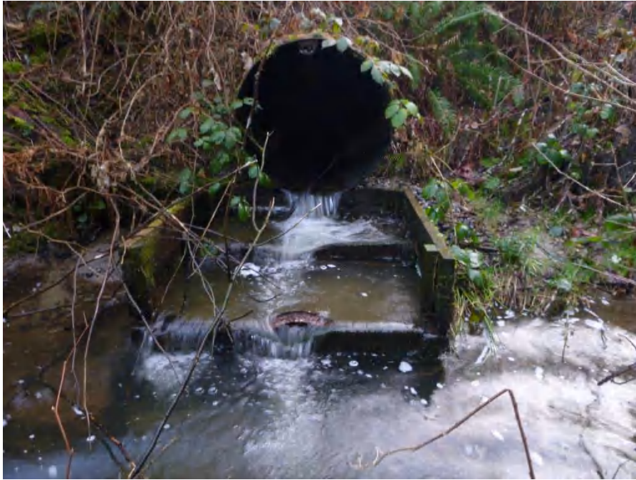
Log weirs placed at the outlet of the first West Bay Road culvert to improve fish passage.
