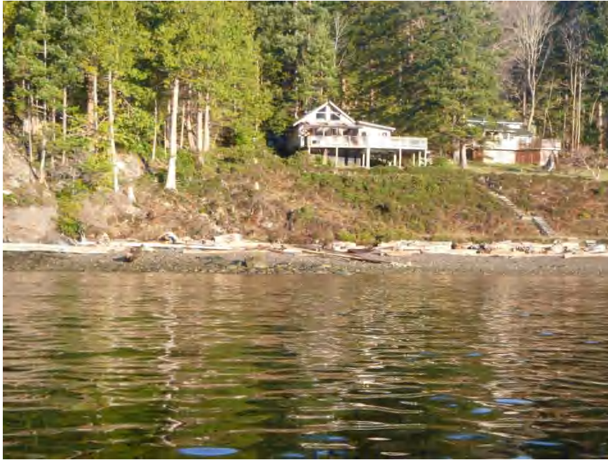
The outlet of Watershed C as seen from the ocean. No outlet drainages were noted. Note the topography associated with the steep ledge.
