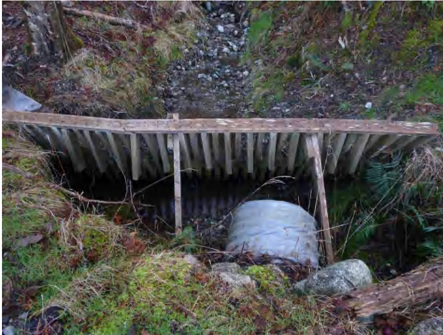
Orchid Creek immediately upstream of the road crossing. Note the wooden grate that was installed to prevent debris from plugging the culvert.
