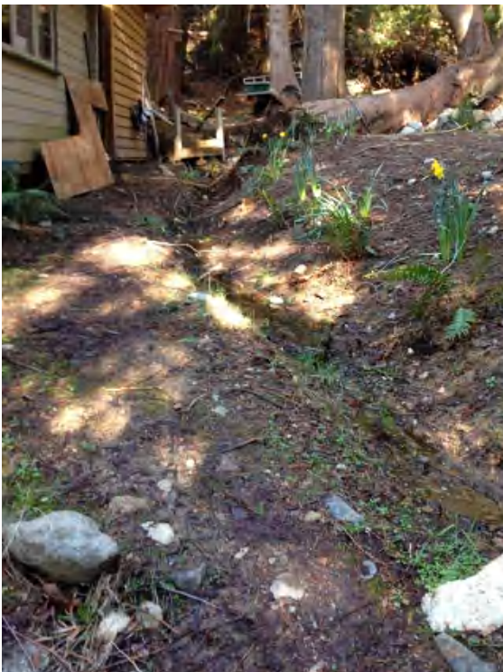
Ditch 2 as it flows adjacent to a house. It should be noted the ditch was manually excavated to ensure water does not inundate the house structure.
