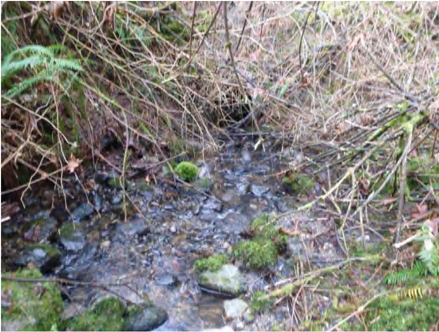
Morphology of tributary 1 upstream of the culvert (barrier) located at the confluence with Grennon Creek.
