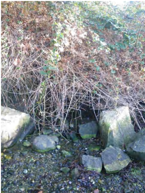
Outlet of the main outlet ditch over a steep (70%) slope to the north of Keats Road.
