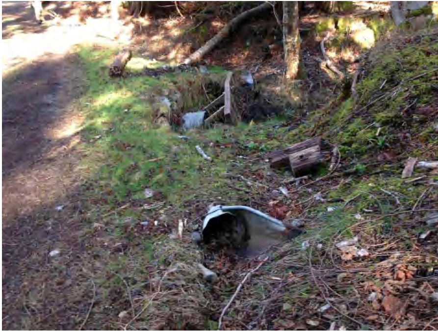
Looking northwest at the area where Ditch 3 flows into Ditch 2.
