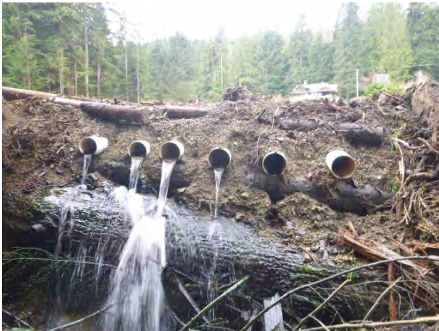
Outlet of constructed dam creating a complex of ponds on tributary 1.
