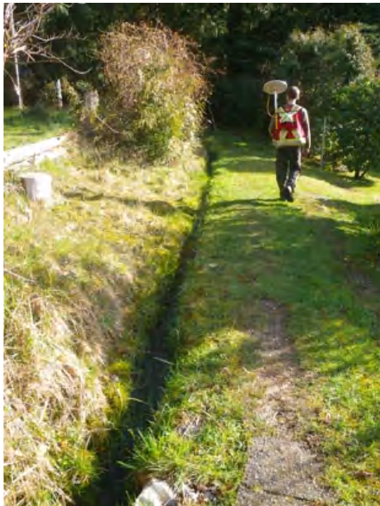
Looking east (upstream) along the watershed outlet drainage upslope of the point where it flows under the access road.
