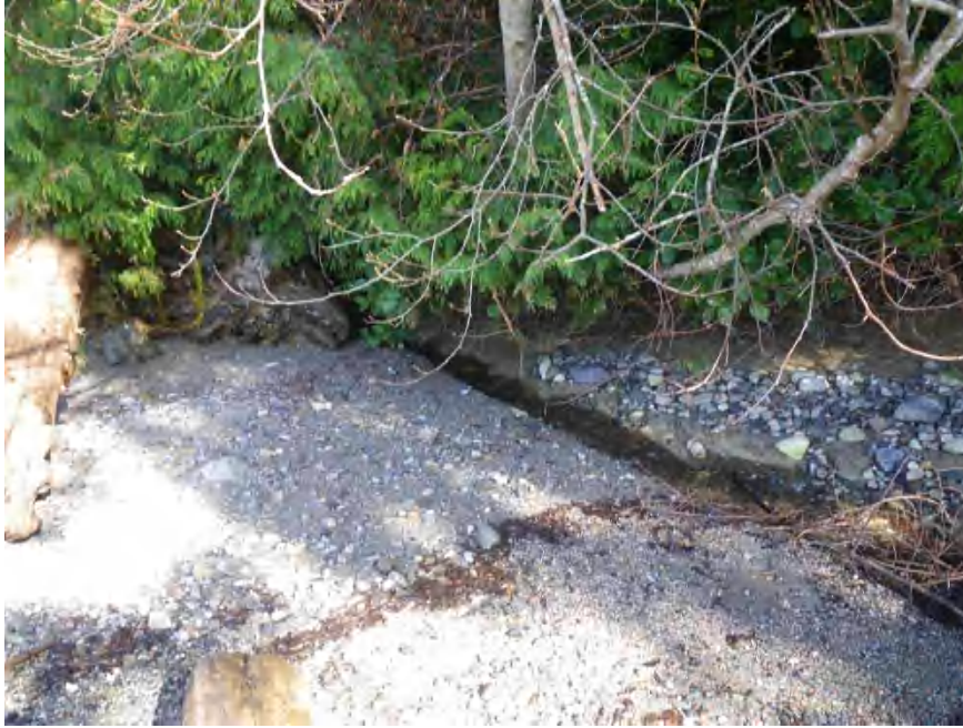
The outlet of Plumper Creek over a gently sloping gravel/cobble beach.
