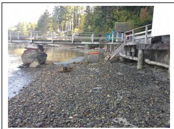
Foreshore structures impeding sediment delivery and flow along beach surface. Photo: RC de Graaf
