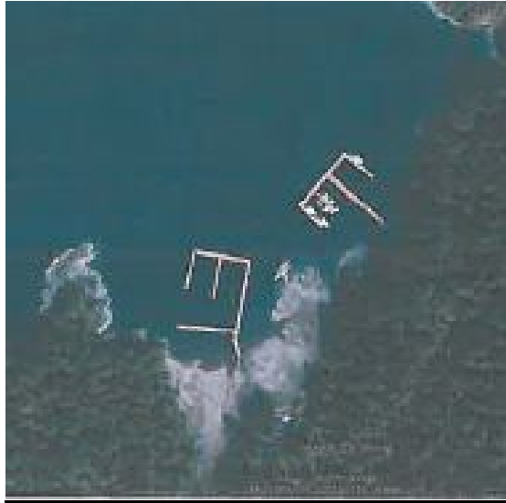
Figure 3. Aerial photo of existing dock infrastructure.
