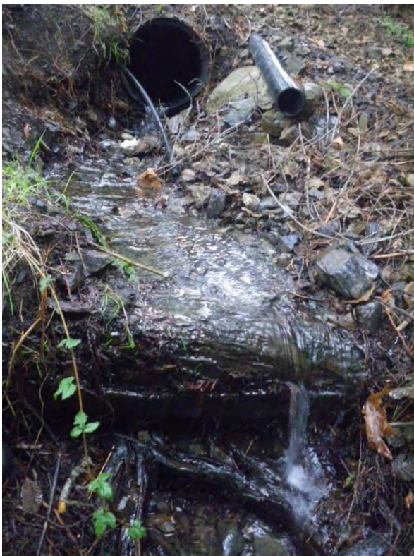
Outlet of the 50 m-long culvert located immediately above the steep slope shown in the previous two photos.
