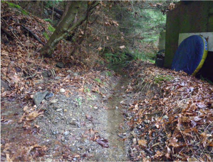
Drainage ditch collecting water from the slope above contributes to flow in the outlet drainage.
