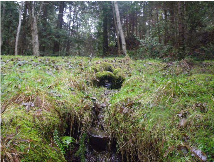
Outlet of the culvert carrying the drainage under the gravel road.
