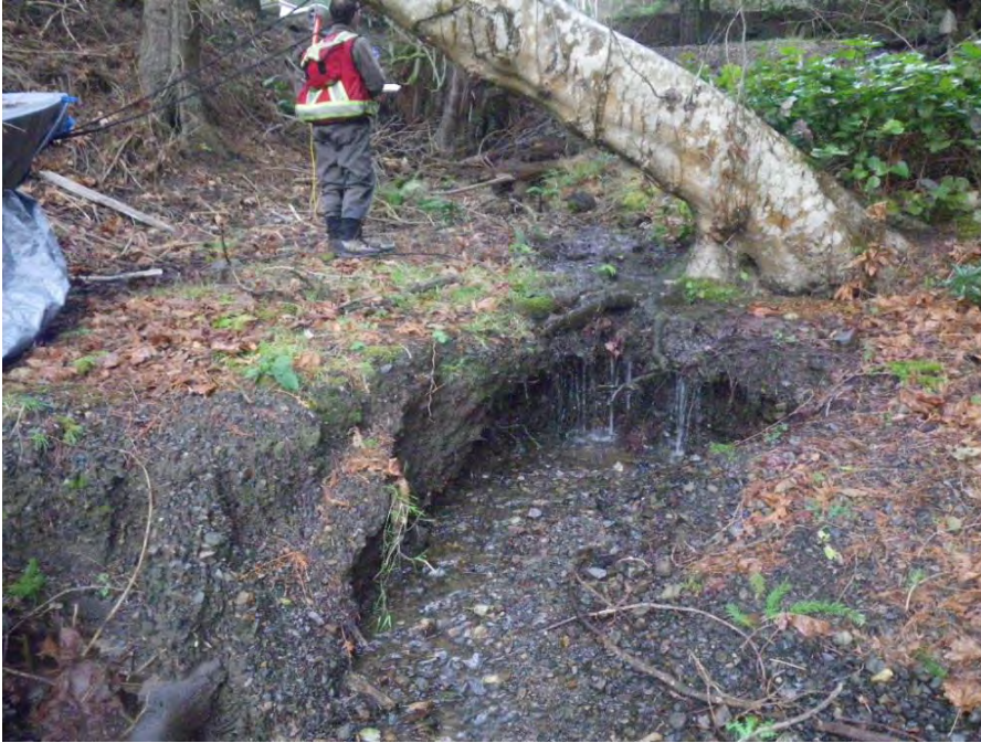
The outlet drainage at the point where it spills out onto a cobble beach at tidewater.
