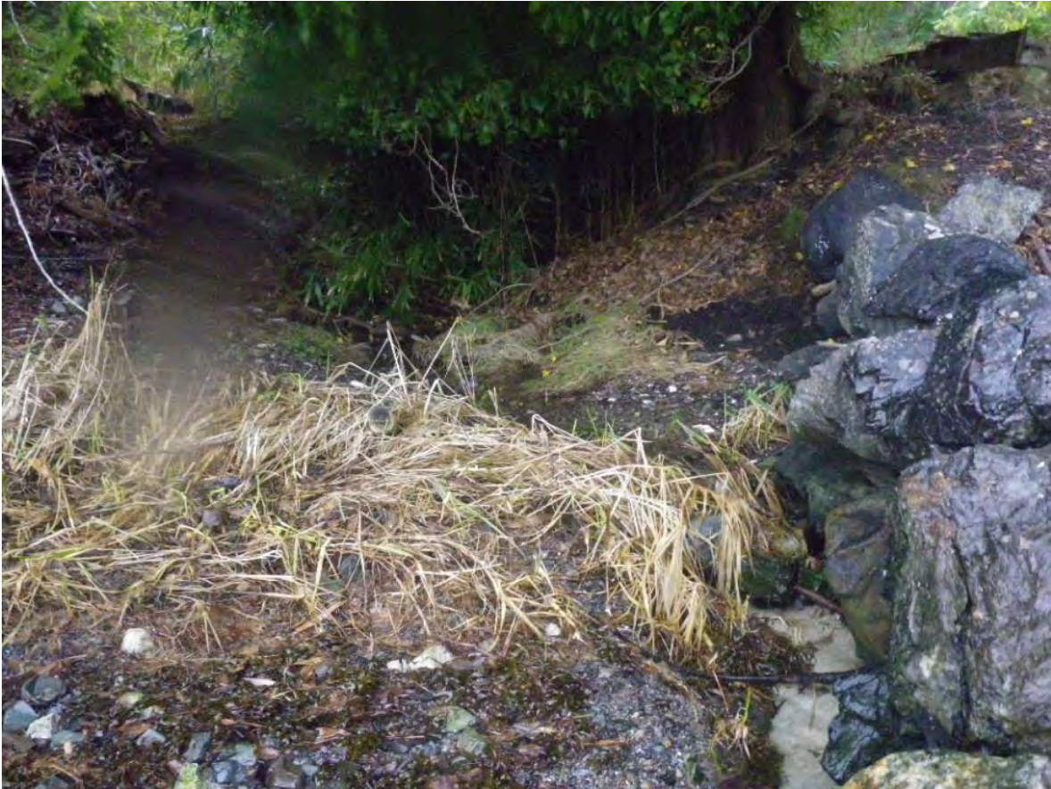
Looking east at the point where the outlet drainage spills out onto the intertidal zone.
