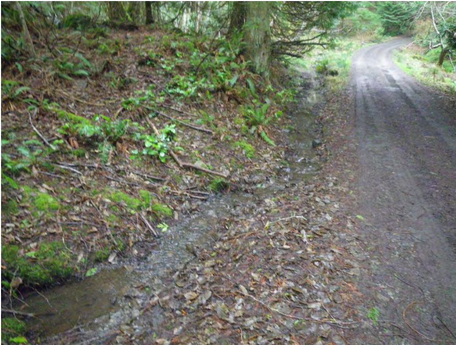
Ditched segment of the main outlet drainage along the gravel road.
