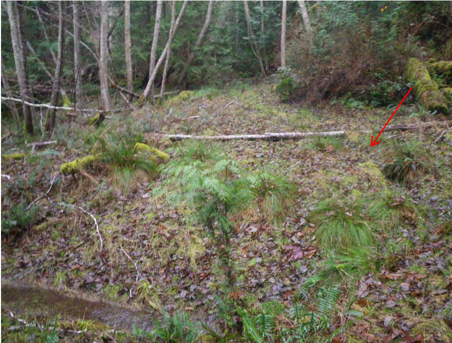
Secondary drainage (highlighted) meeting the main ditched segment of the outlet drainage close to the inlet of the culvert under the gravel road.
