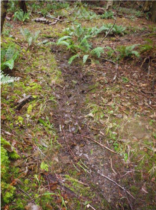
Poorly defined characteristics of the outlet drainage upslope of the gravel road crossing.
