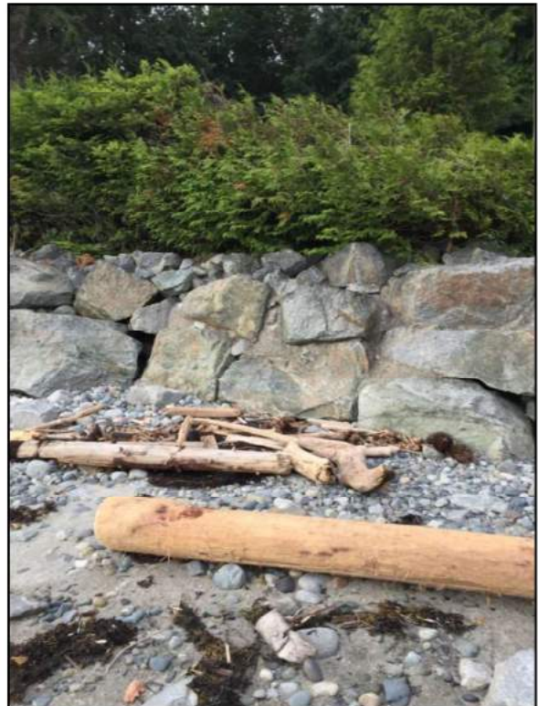
Photograph 2 – Rip Rap Revetment
