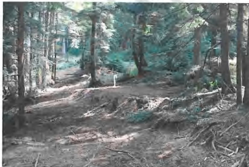
Figure 9: Existing septic system, facing north-east
