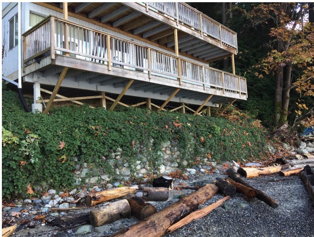
Figure 1 Existing dwelling and rock retaining wall
