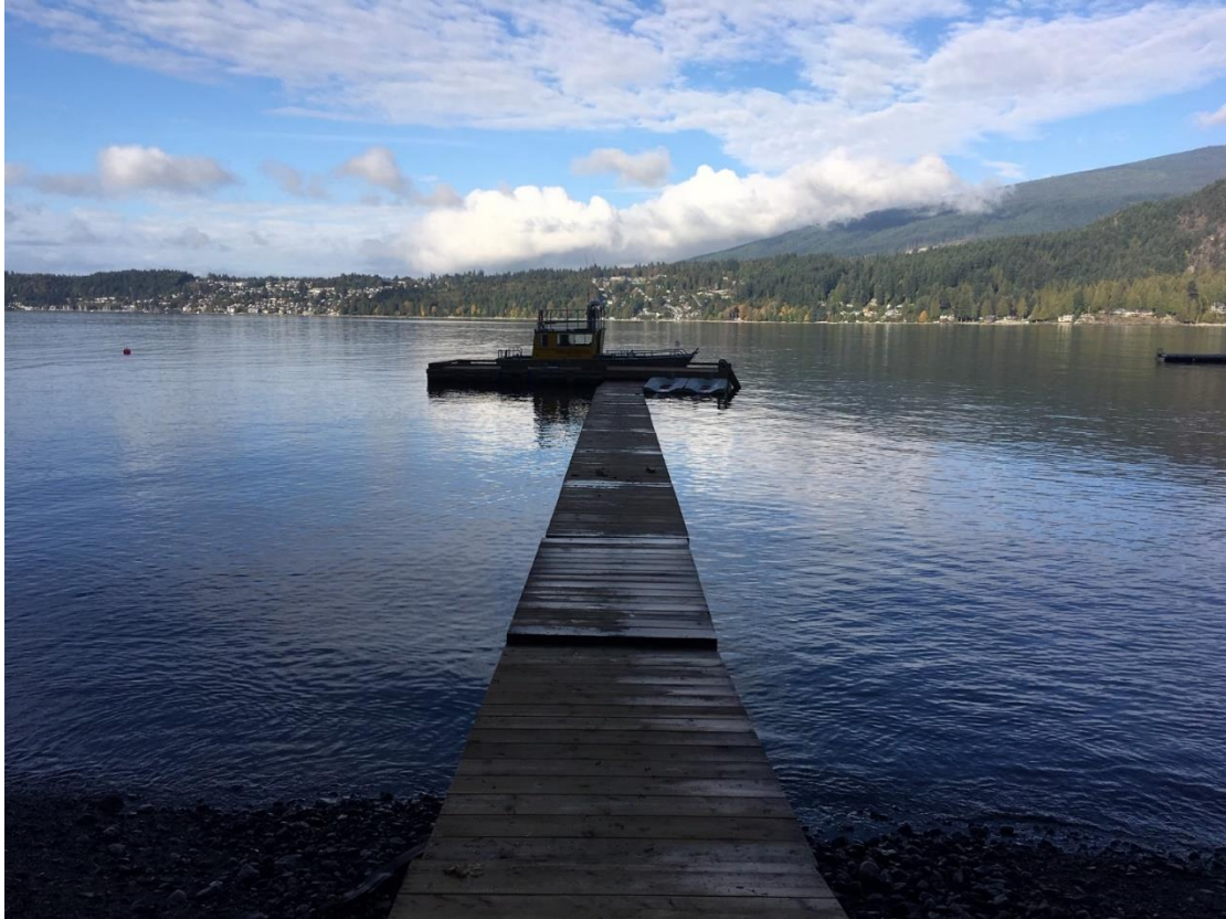
Figure 2 Existing dock and float structure
