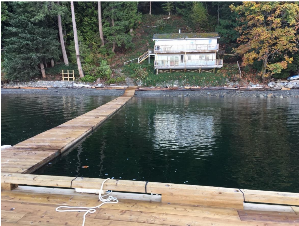
Figure 3 Existing dock and float structure
