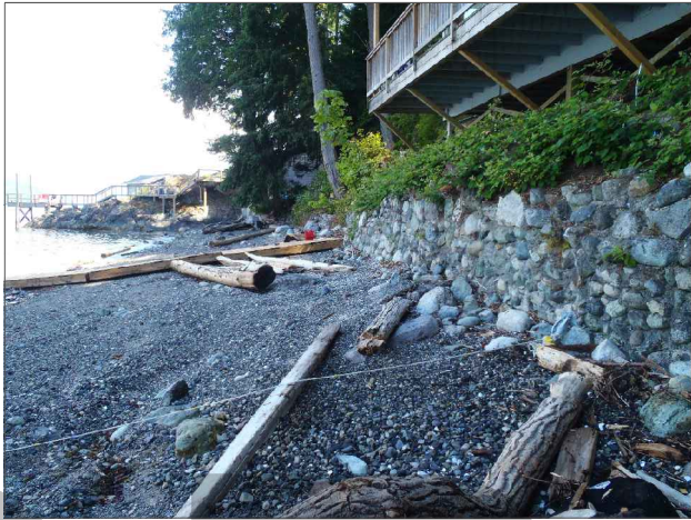
Photo 2. Property retaining wall and shoreline. View looking north.
