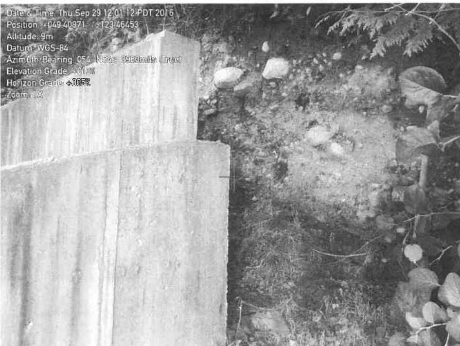
Waypoint 6. Concrete retaining wall supporting cutslope, Lot 14.
