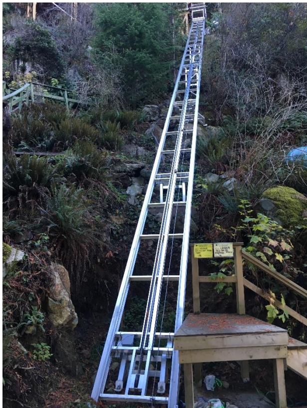
Figure 3. Existing Tram Structure
