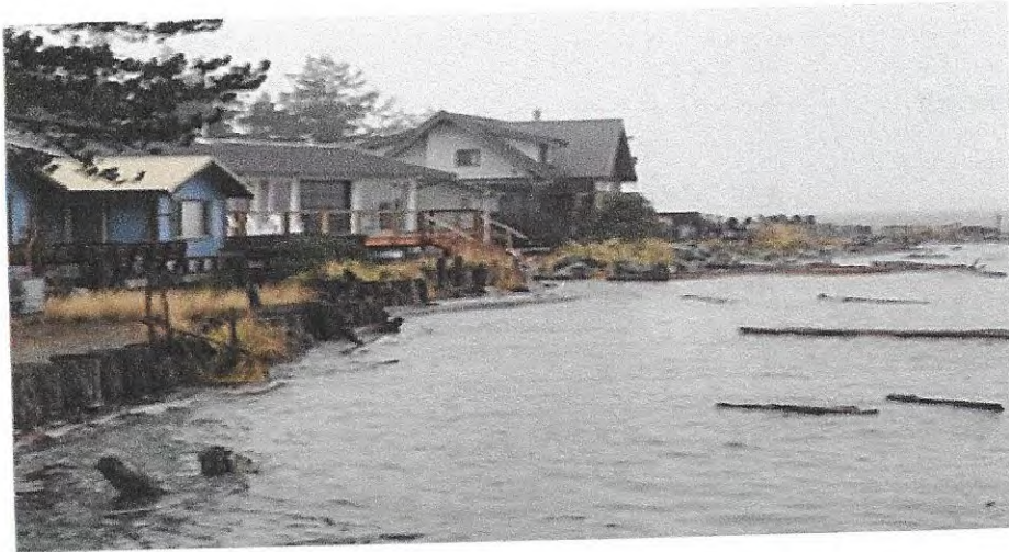
Vaucroft, view from SCRD wharf looking north, December 27, 2022. Properties north of wharf (Lots 1, 2 and 3) protected by seawalls.
