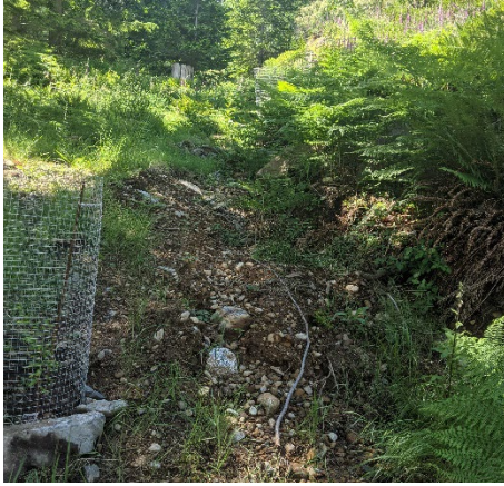
View of the shallow constructed channel #2 along the slope base
