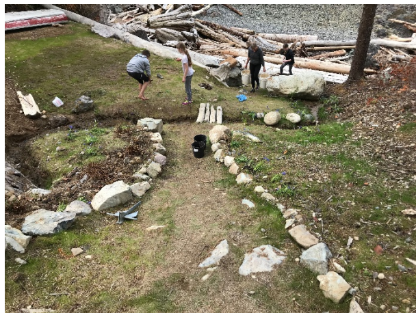
View of constructed channel shortly after construction (provided by the owner).
