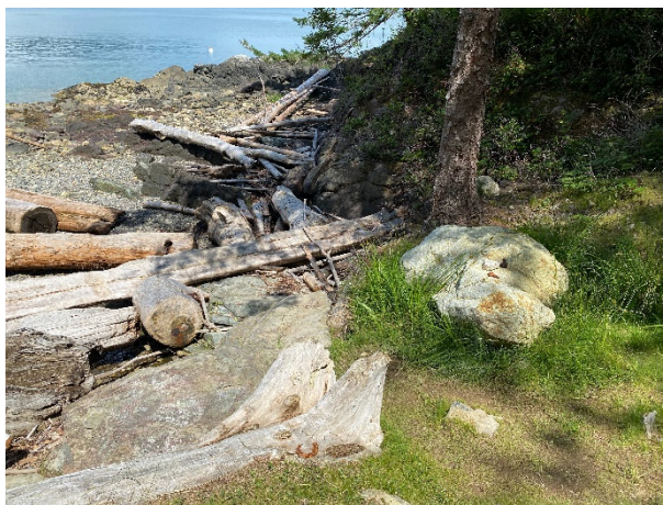
View of the constructed channel outlet onto the beach (provided by owner).
