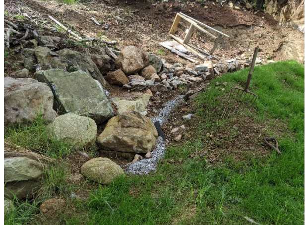
View of the buried drain tile around the upper bench.
