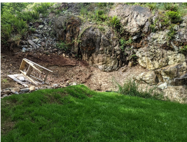
View of the upper bench during the site visit.
