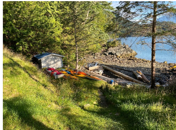
View of the trench post construction (provided by owner).
