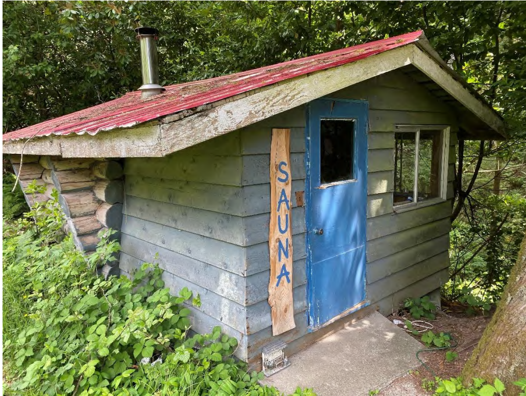
Accessory building (sauna)
