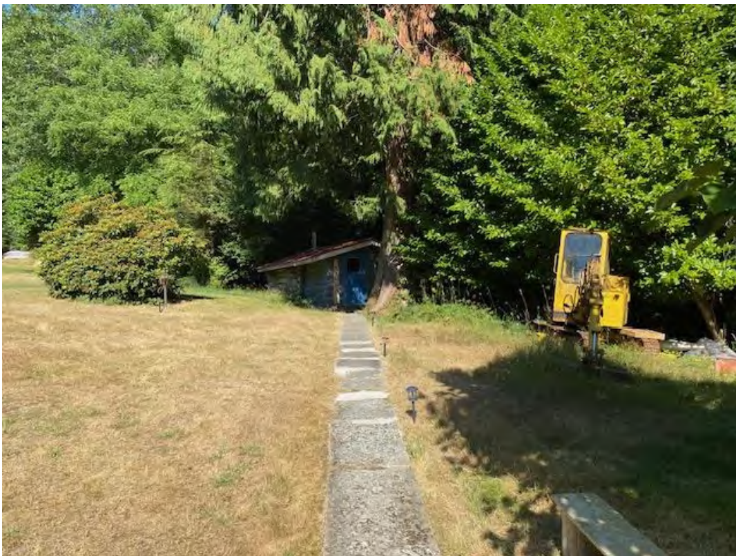
Accessory building (sauna)
