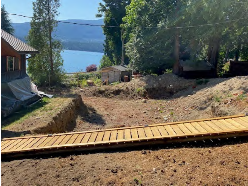
Photo 3: View from east side lot line.
