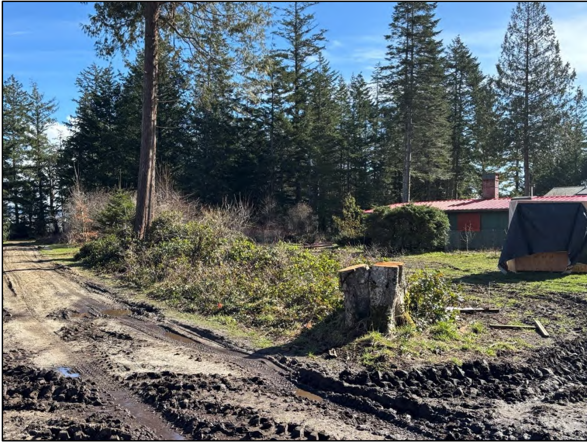
NORTHERN PROPERTY LINE AND BUILDING SITE, LOOKING EAST
