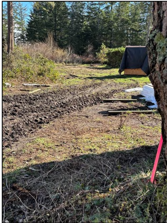
NORTHERN PROPERTY LINE AND BUILDING SITE, LOOKING EAST
