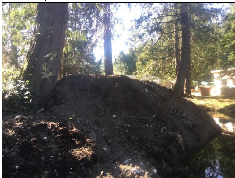
Figure 7, Image of spoil pile beside pond that abuts a cedar tree. Regrade base of tree, spread material and replant regraded area with native vegetation or legume mix.
