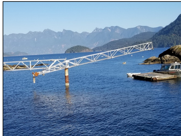
Photo 5. Site 7 float and gangway.
