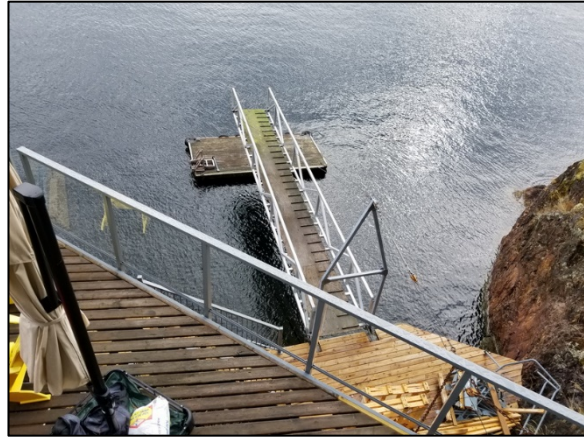
Photo 3. Site 4 float and gangway.
