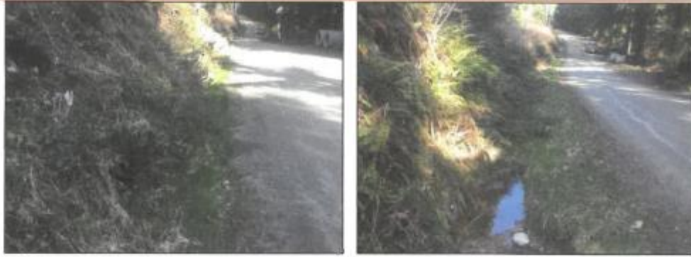
a b Figure 3, view of West Bay road ditch along Lot 80. Photo (a) is the view northeast from the south corner of the property. Photo (b) is view to northeast from the driveway location. The ditch is shallow (<20cm deep) indicating a low volume of water.
