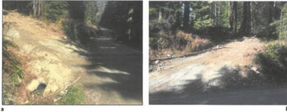
Figure 6, A rough driveway had been installed prior to the assessment. Photo a is view to the southeast showing the culvert. Photo b is the view up the driveway.
