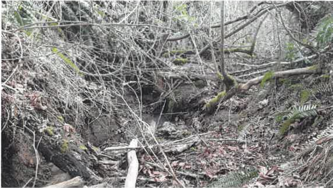
Photo 4: Looking downstream/south at the culvert crossing for No Name Creek. March 5 th , 2019
